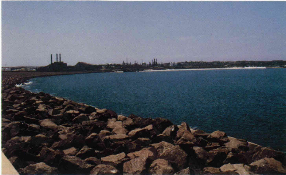
Figure D6.3 A Conventional Two-Layer Armoured Seawall
