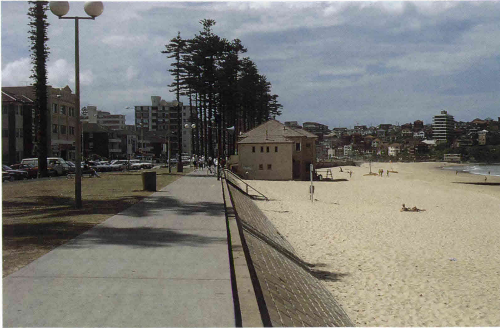
Figure 5.3 Seawall and Promenade, North Steyne, Sydney.
