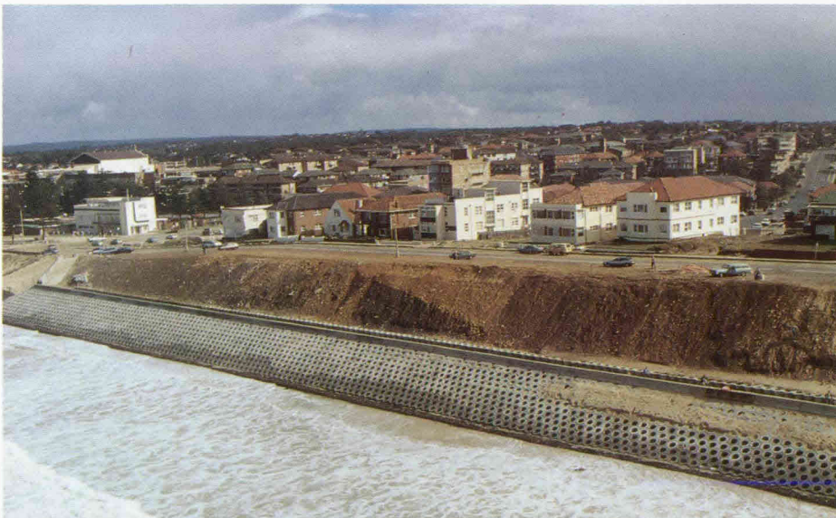
Figure D6.1(d) Semi-rigid Seawall of SEABEES®
