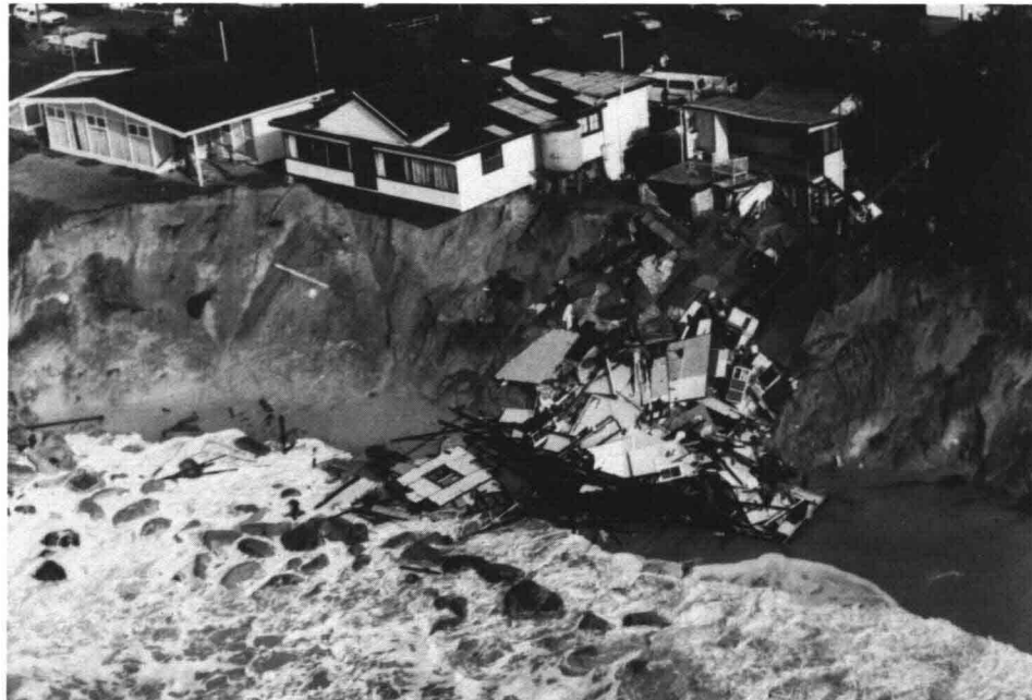
Figure C2.1 Undermining and Collapse of Buildings Caused by Beach Erosion
