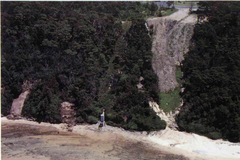
Figure C7.2 Landslip Failure of Coastal Bluff, Bateau Bay, Wyong Shire
