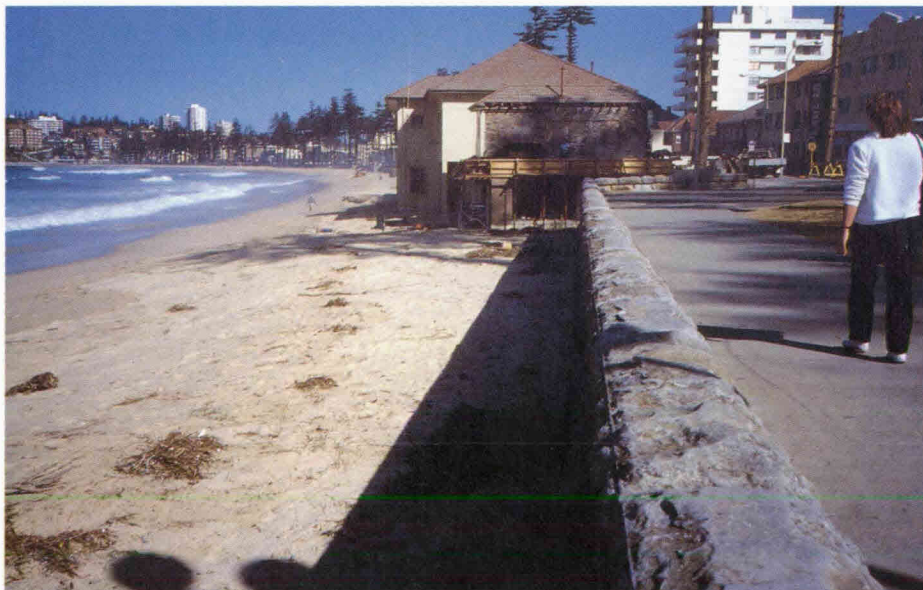
Figure D6.1(a) Rigid Vertical Seawall
