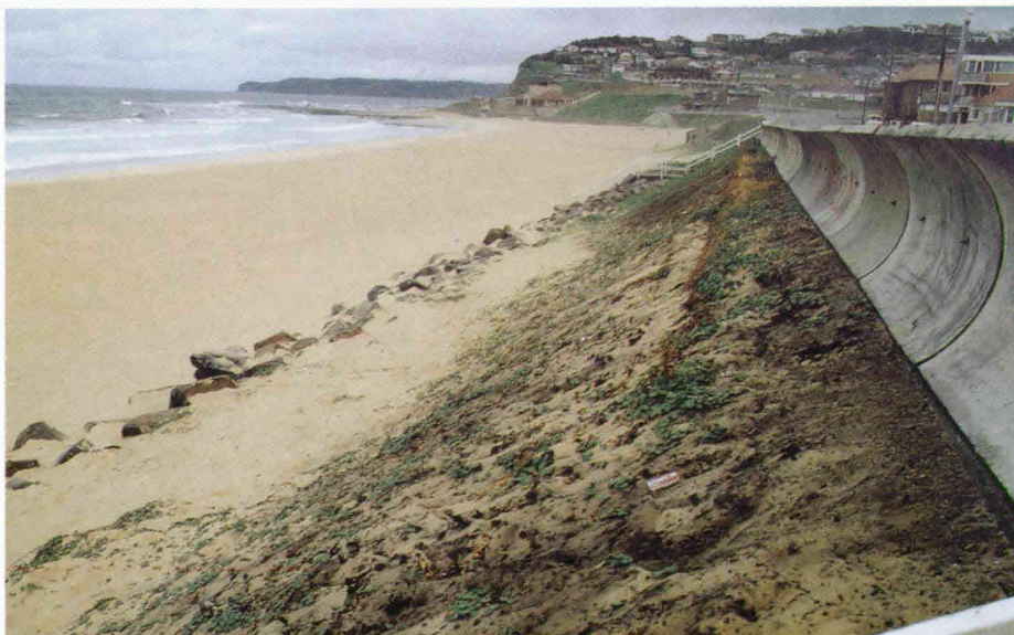
Figure D6.2 Curved Wave Deflection Barrier on Crest of Seawall
