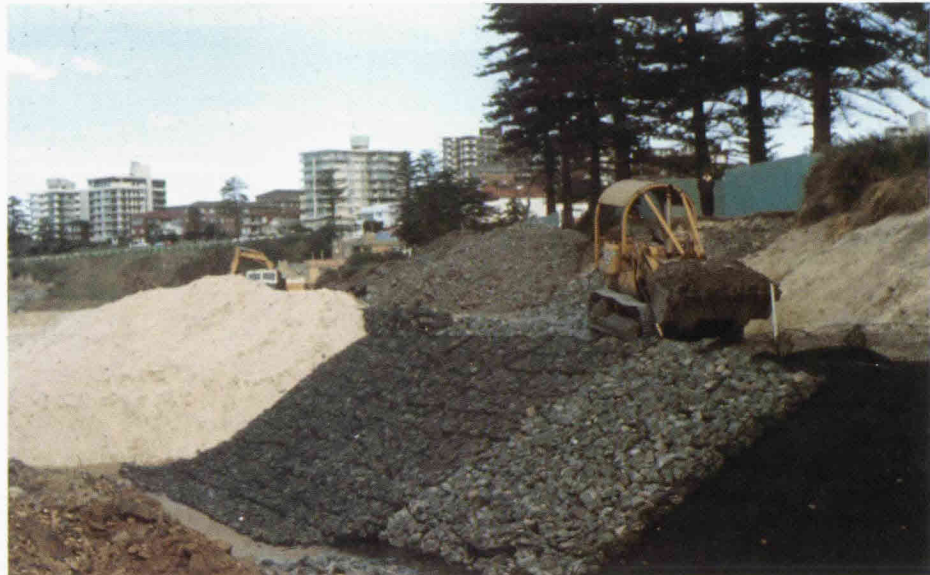
Figure D6.1(c) Sloping Gabion Seawall
