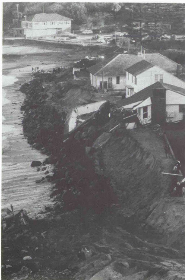
Figure 5.5 Severe Beach Erosion, 1974 Storms, Bilgola Beach, Sydney.
