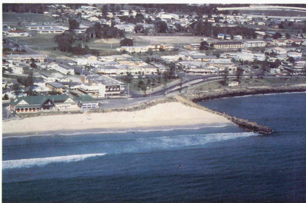
Figure 5.4 Groyne Structure, Kirra Beach Qld.
