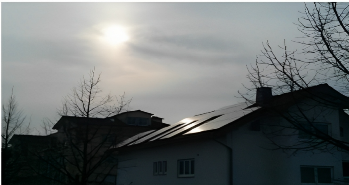
Figure 1.1: PV system on Private House in Hangelar, Germany [4]
