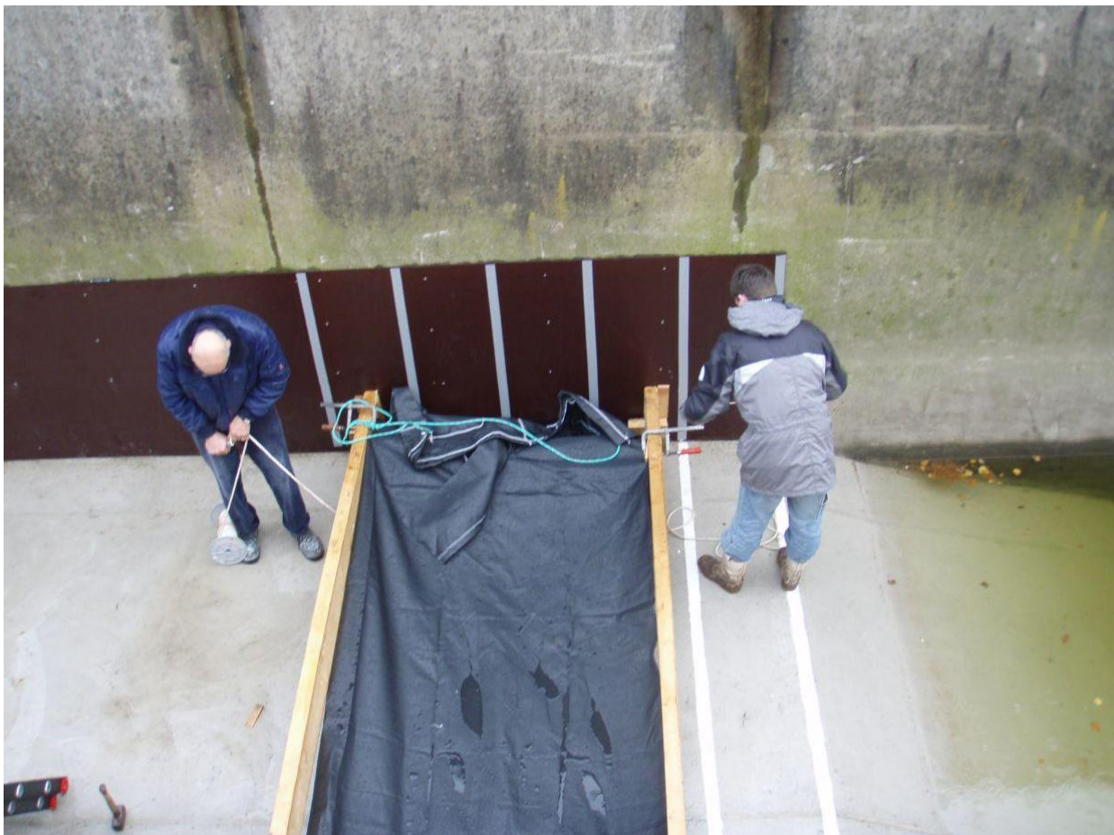
Photo 10: Lay out geotextile tube
