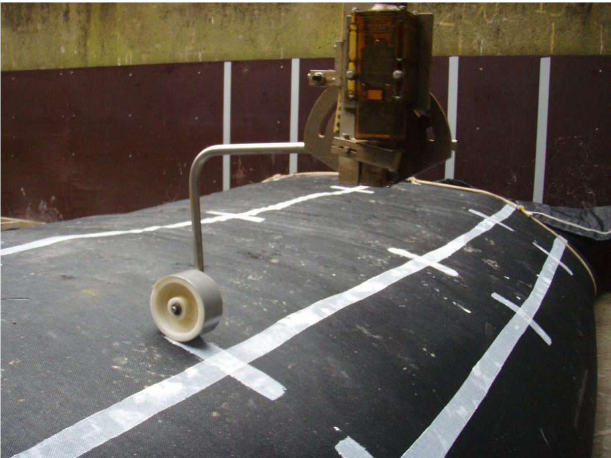
Photo 22: Profiling geotextile tube
