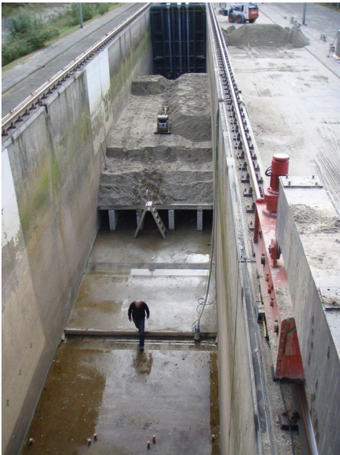
Photo 6: Building the sand core
