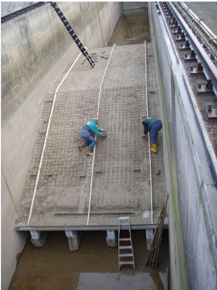
Photo 8: Installing the reinforcement
