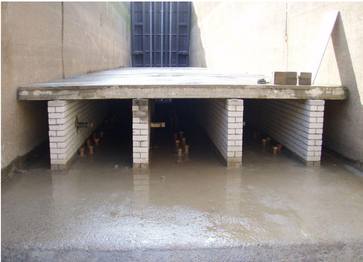
Photo 4: Back flow structure
