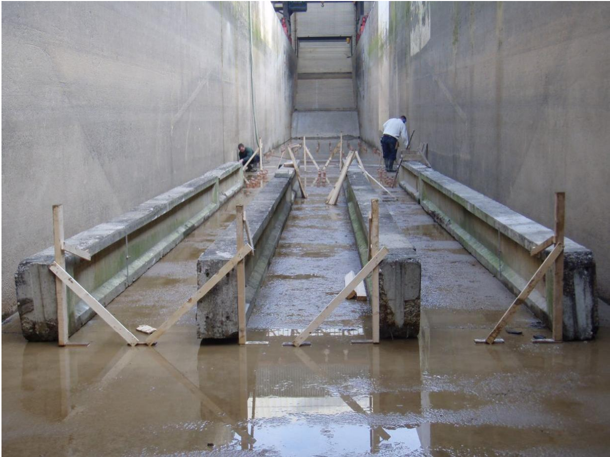
Photo 1: Lining out the Back flow structure
