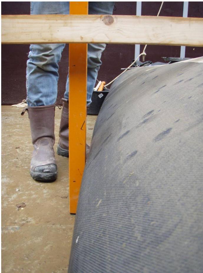
Photo 24: Determine outermost point geotextile tube
