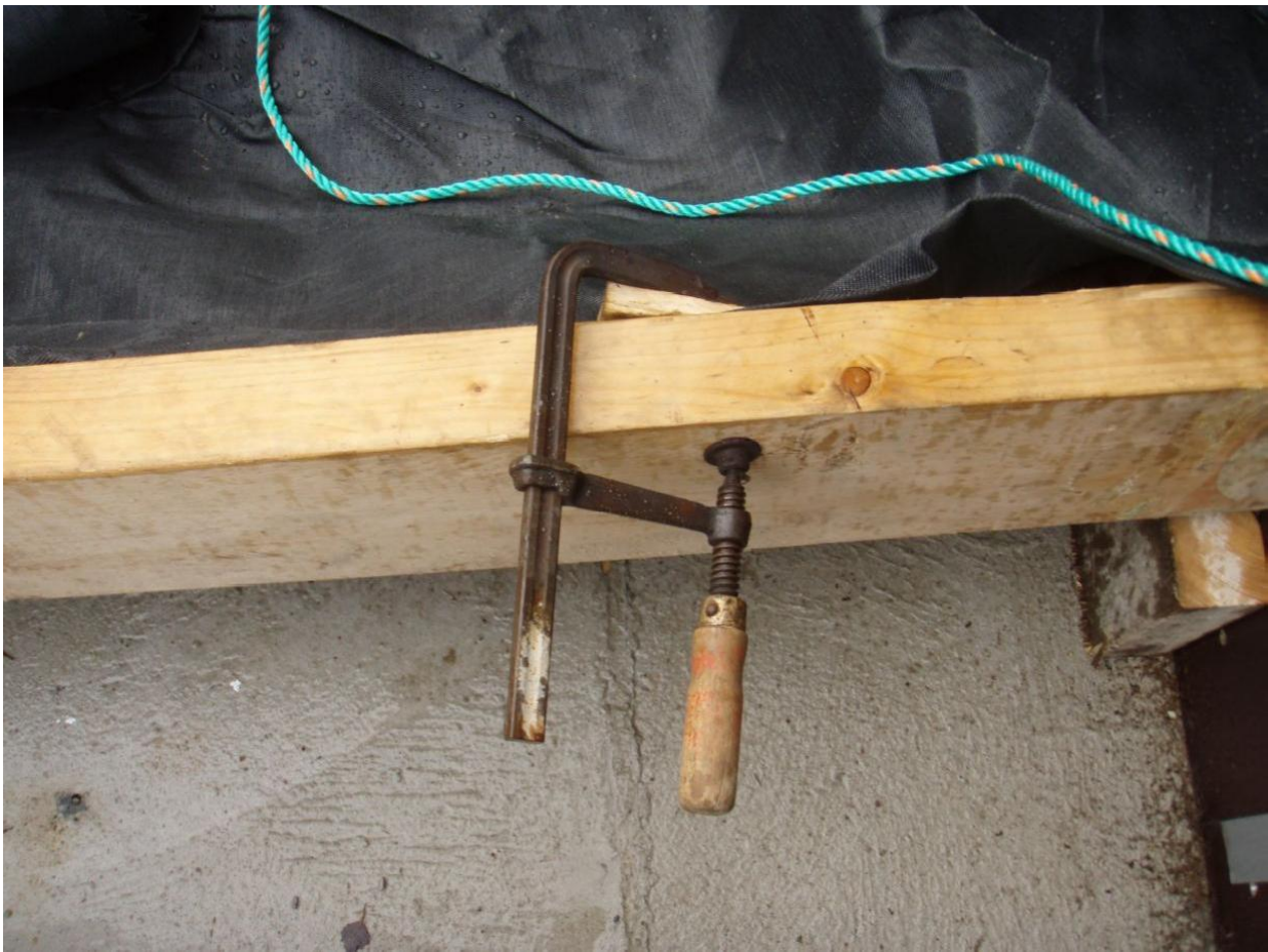
Photo 11: Temporarily fixation geotextile tube
