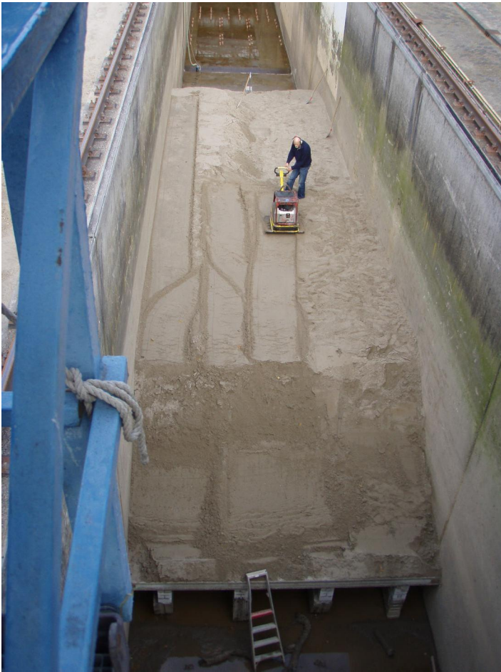
Photo 7: Compacting the sand core
