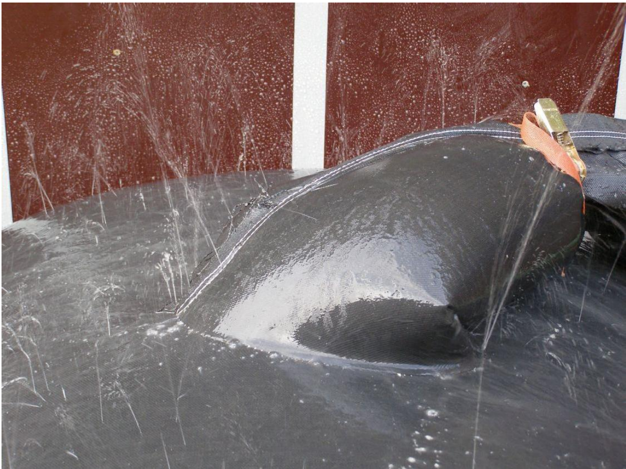
Photo 16: Process water flows through the geotextile during filling
