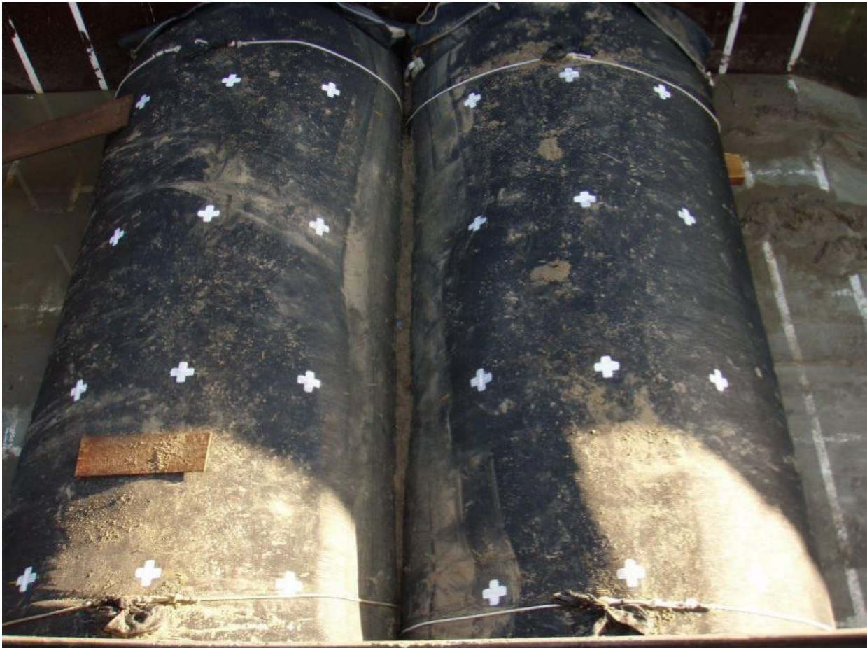
Photo 45: Prepared geotextile tubes before test series P2-1
