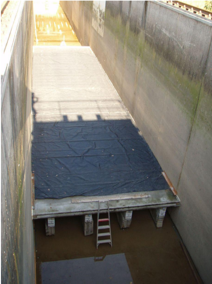
Photo 5: Geotextile on the concrete plates to avoid erosion
