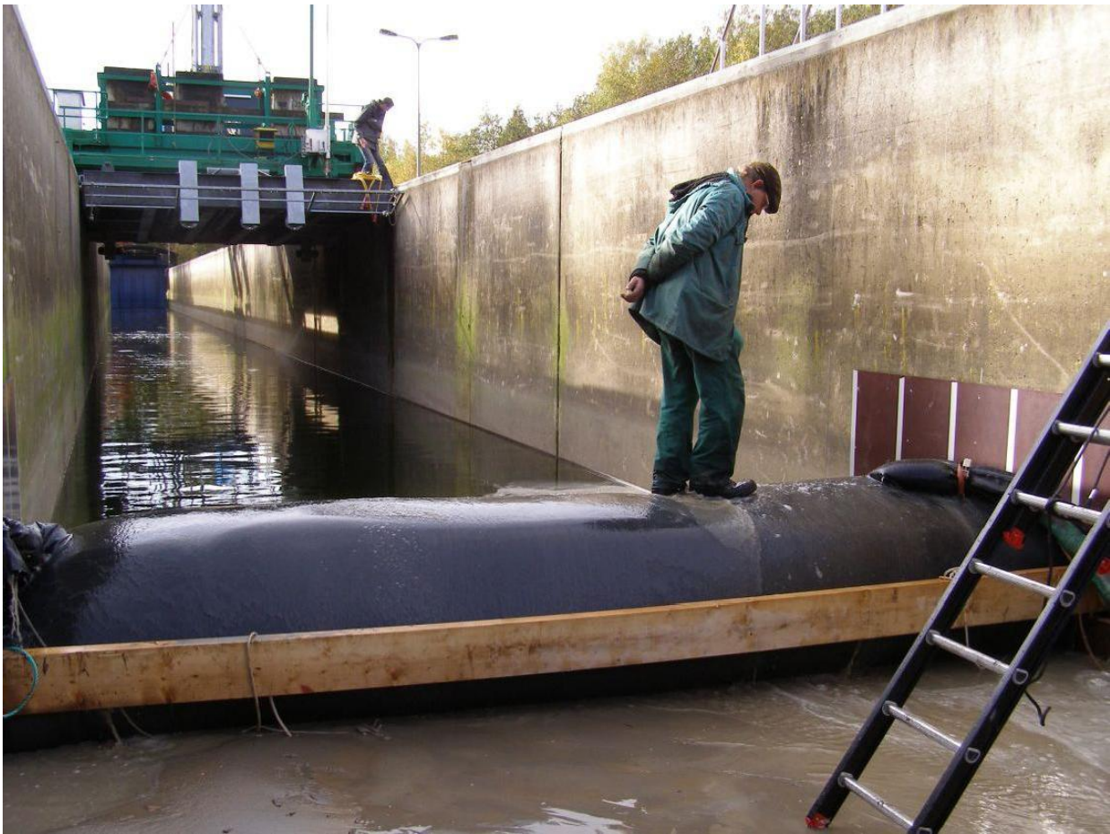
Photo 15: Walking over geotextile tube to prevent blocking
