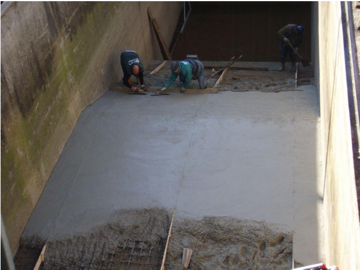
Photo 9: Application of the concrete
