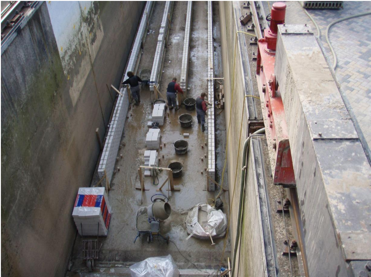
Photo 2: Building the Back flow structure
