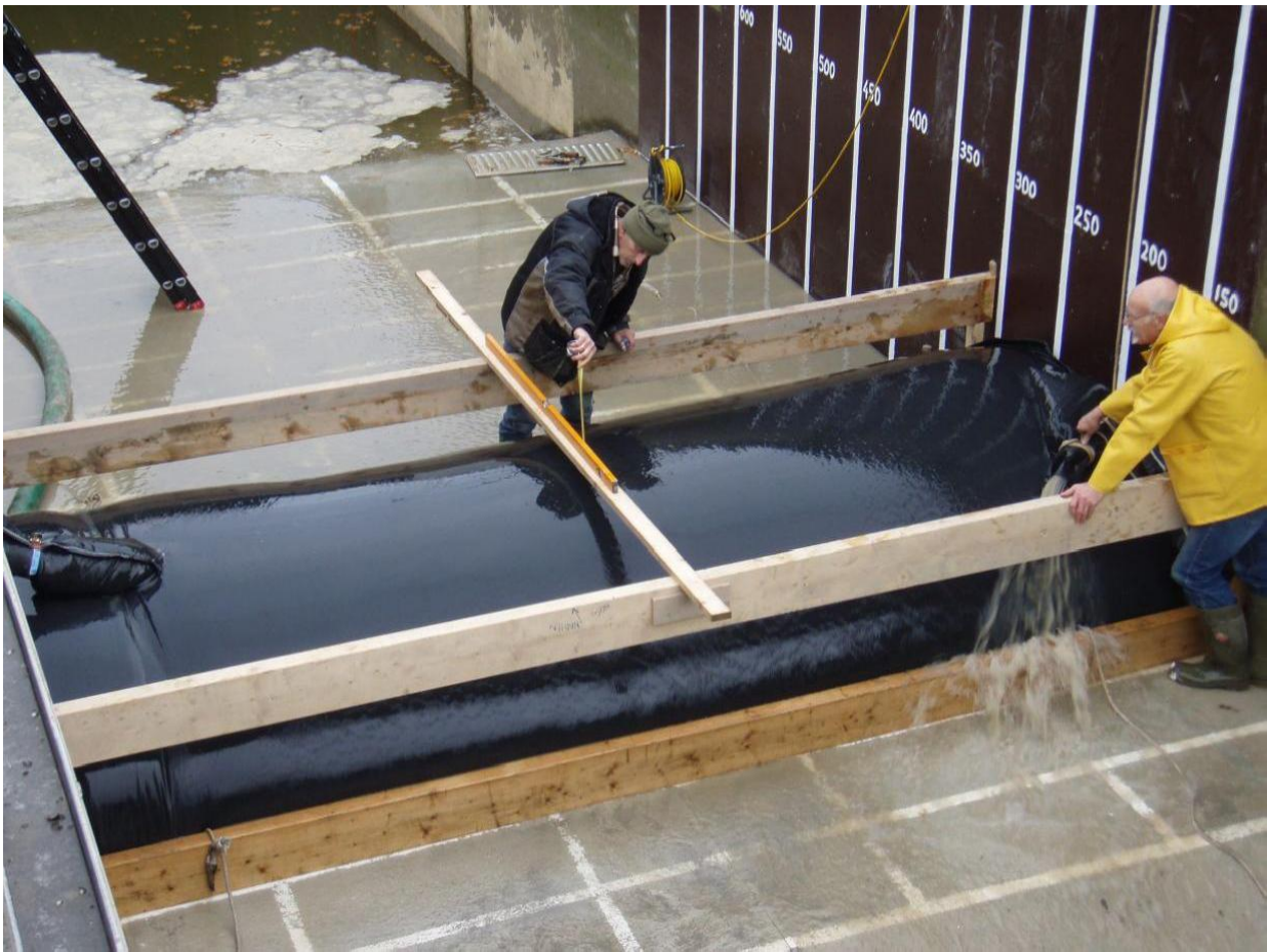
Photo 13: Filling the geotextile tube and measuring the actual height
