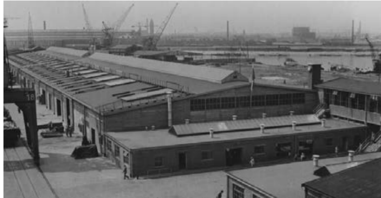
Demolish and rebuild into a design and innovation building
