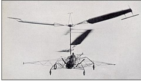
Figure 2.2: Corradino d'Ascanio's helicopter with servo tabs.
