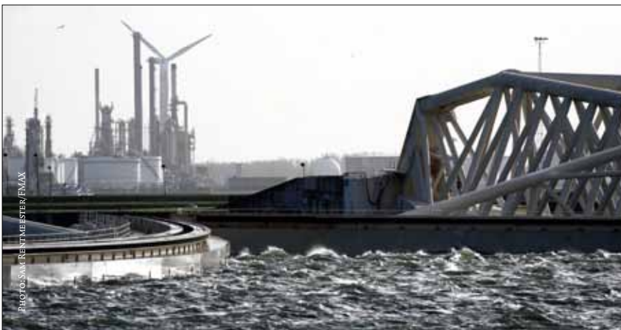
The Maeslant storm surge barrier at Hoek van Holland.
