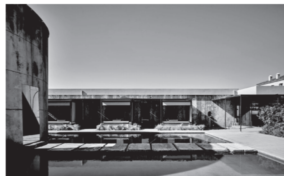
Concrete blocks divided for wine storage tanks (5m x 6m) used as hotel rooms. Doorway openings - slabs used as stepping pathway.
