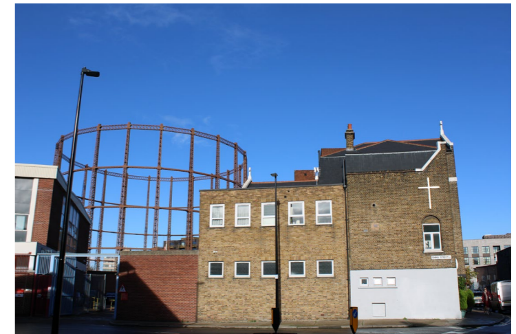
View from Hackney Road The lightweight structure of Gasholder No.5 seen in the background gives a glimpse of the industrial heritage of the area while contrasting with heavy brick building in the foreground.
