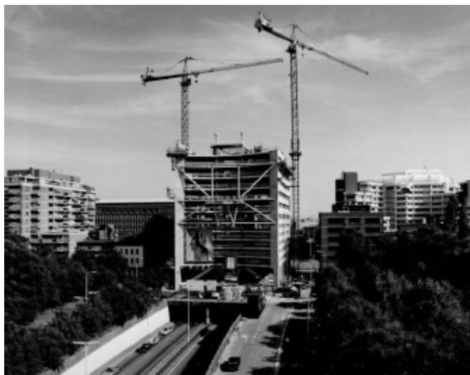
Fig. 1. Construction of the Malie Tower in The Hague
