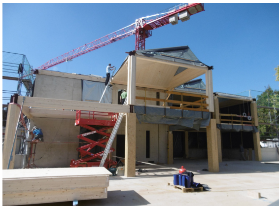
Figure 8. Assembling building on site (Wächter + Wächter Architekten, 2019)
