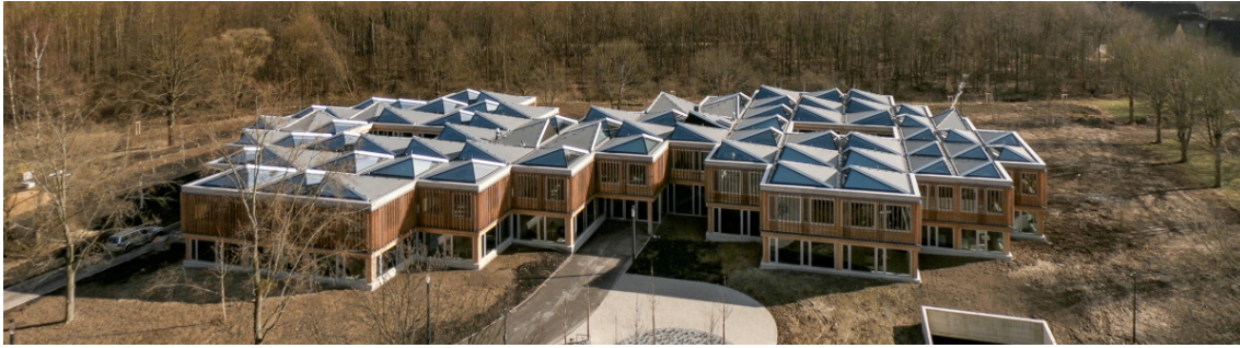
Figure 7. AIZ campus Kottenforst (Waechter + Waechter Architekten, 2019)
