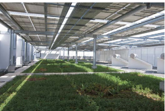
Figure 9.31- Rooftop green roof and solar panels (DEWA HQ, Dubai) Source: www.constructionweekonline.com/
