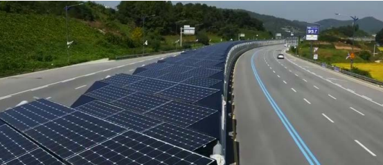
Figure 9.46- Solar panels in road buffer used as a covering for bicycle paths
