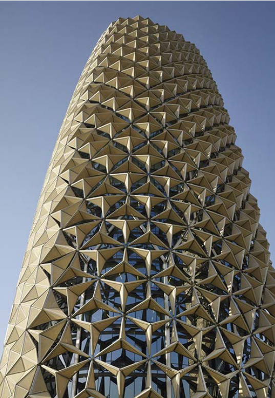
Figure 9.49- Facade cover on Al Bahar Tower, Abu Dhabi (right) Source: https://www.e-architect.co.uk/dubai/al-bahar-towers-abu-dhabi
