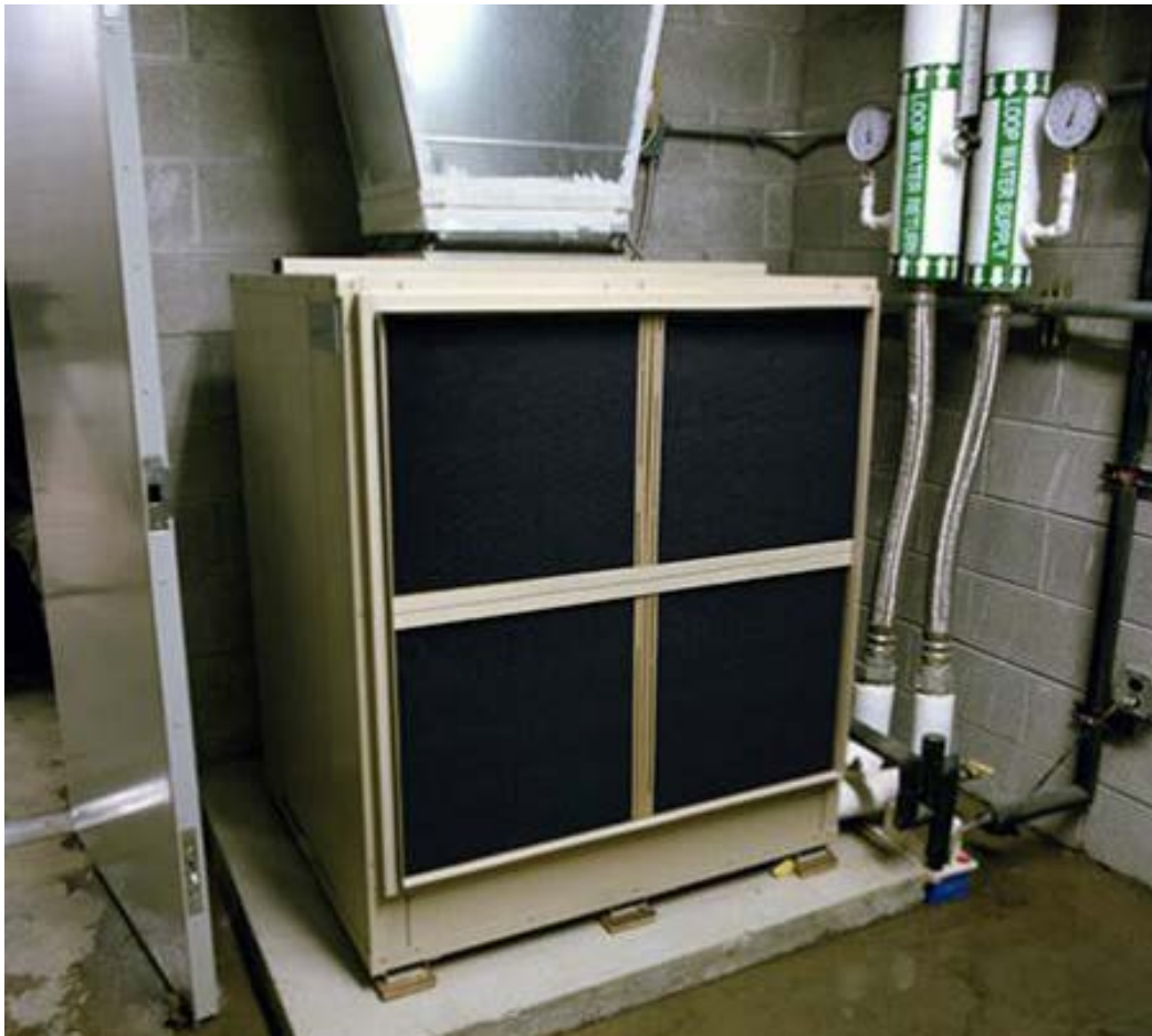
Figure 8.36 - A commercial-scale ground source heat pump system. Source: Craig Miller Productions, NREL
