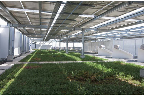
Figure 9.48- Rooftop green roof and solar panels (DEWA HQ, Dubai) Source: www.constructionweekonline.com/
