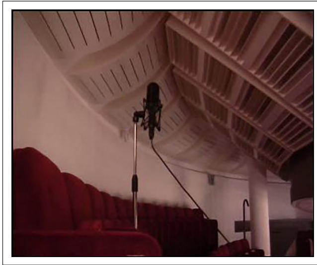
Figure 12. Measurements in the gallery with acoustic panels on the ceiling.
