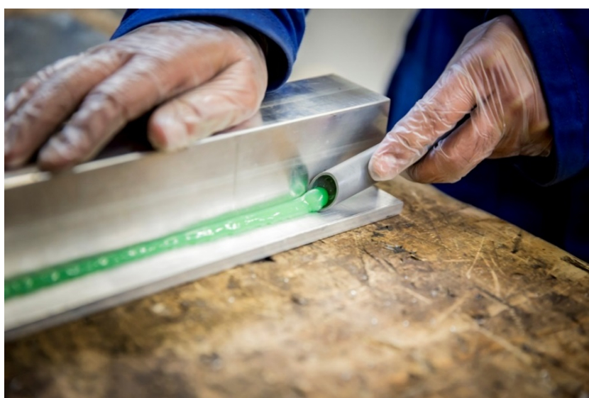
Figure A.80: Finishing of bondline
