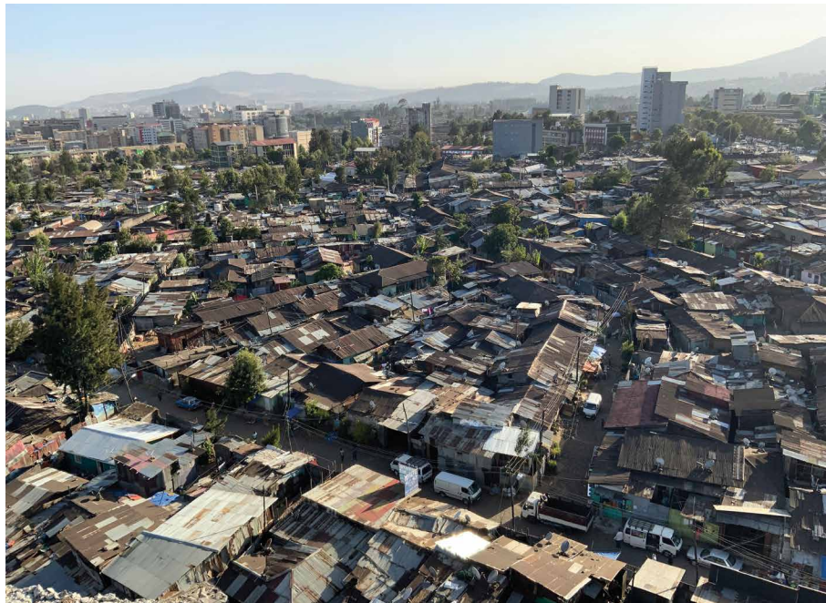
FIG. 2.7 Areal view of sefer with the characteristic pockets of spaces, narrow alleys, and rusty, corrugated iron sheet roofing.
