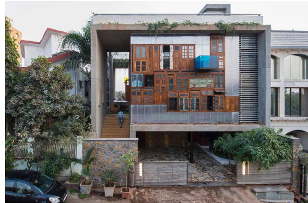
Figure 5.1.3. Casa Collage by S+PS Architects; a project where building components are reused to create a unique facade.
