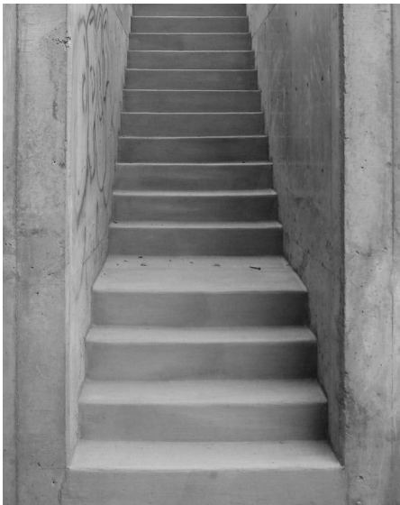
Park Modern: Panel formed, site poured concrete < http://blog.buildllc.com/2014/11/a-visual-guide-to-stairs/ > [Accessed 21 March 2019].
