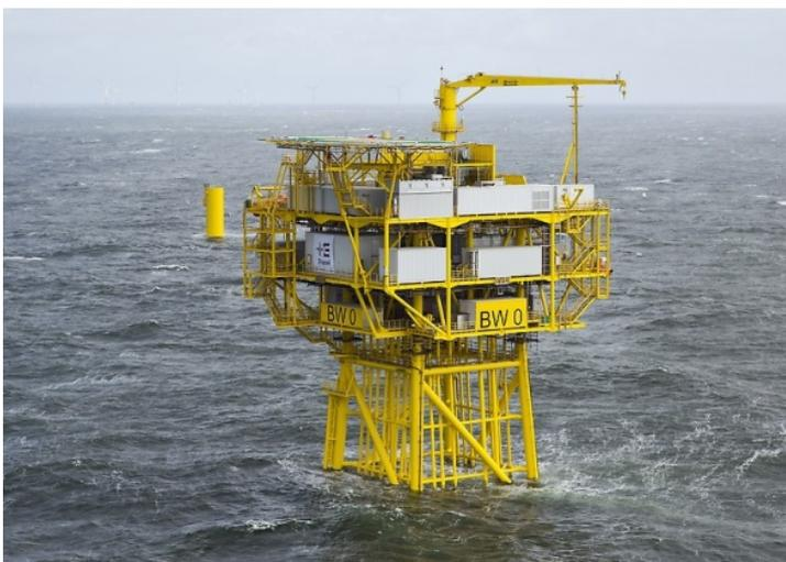
Figure 1.3: Equipment housed in separate encasements (image courtesy of Overdick: <http://www.overdick.com/>)
