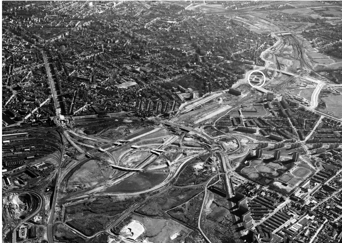
Ring road under construction (ca. 1969)
