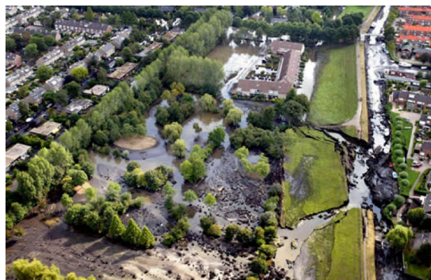
Figure B.1 - Dike breach in Wilnis Source: Middendorp, 2016
