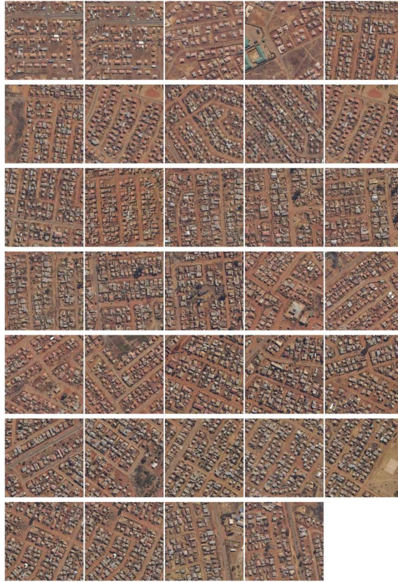
Fig. 34. Cluster A sample images with classification of a mixed architecture and a formal urban design
