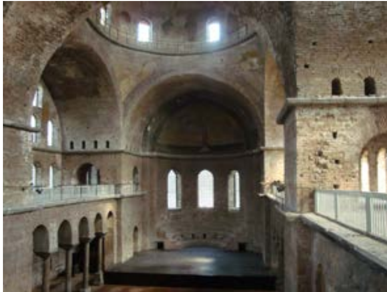
Figure 7 The construction of the Hagia Irene with the dome, thick walls and arches (photo taken by author)
