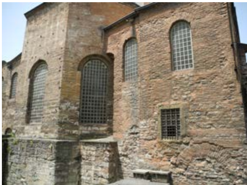
Figure 8 Different kinds of bricks and compositions in the outer part of the east façade at the apsis (photo taken by author)
