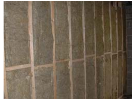
Inside cavity wall: Timber frame
