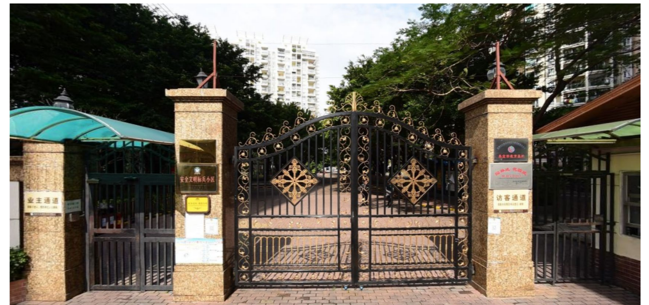
Figure 4-54: Photo of gated commercial housing in Sungang Source: author
