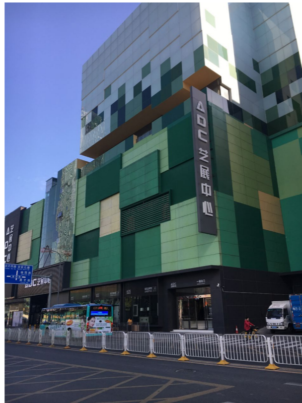
Figure 4-55: Photo of transformed factory compound in Sungang Source: author
