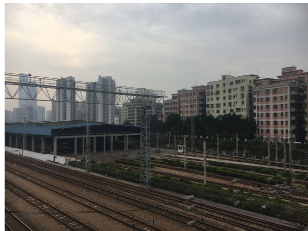
Figure 4-56: Photo of railway tracks in Sungang Source: author
