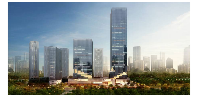
Figure 4-7: Image of pilot project "Zhaoshangzhonghuan" in Luohu District from Luohu government Source: Luohu, n.d.
