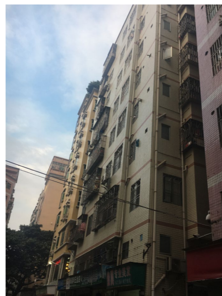
Figure 4-53: Photo of urban village in Sungang Source: author
