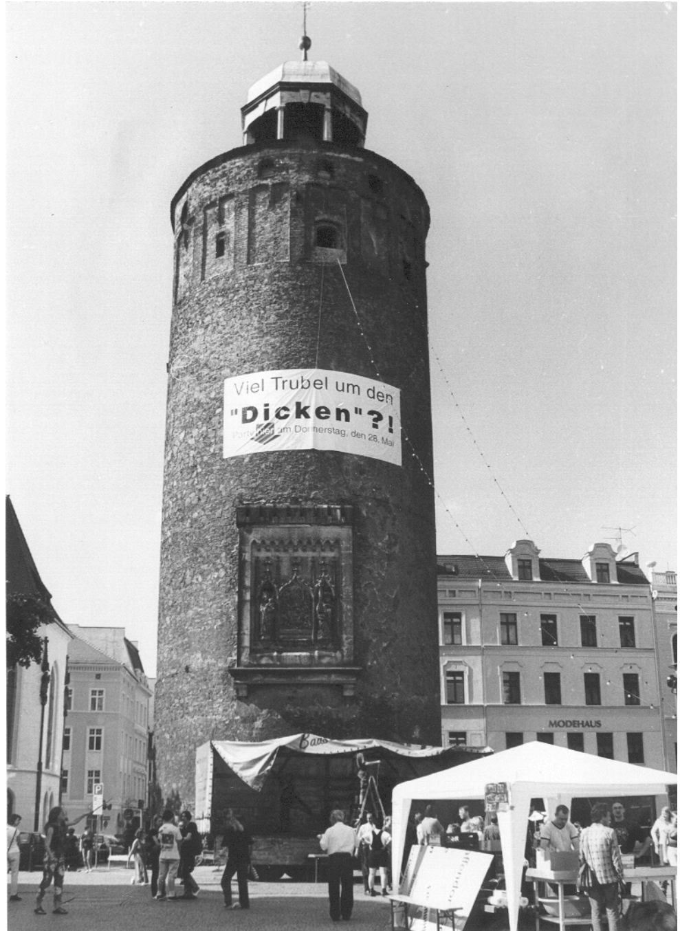
Fig. 17. Dicker Turm during the 1998–99 restoration campaign, showing the banner “Viel Trubel um den Dicken” and temporary stands in front of the tower. From the Sammlung Brettschneider, shared by Siegfried Hanzl on Facebook, 28 July 2024, original source unidentified.
