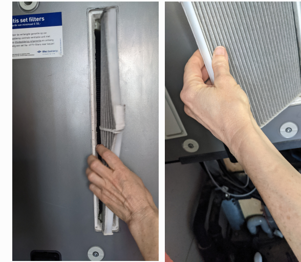
Fig. 35: Inconvenient to change filters of MVHR unit
