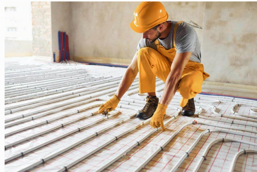
Fig. 8: Underfloor heating
