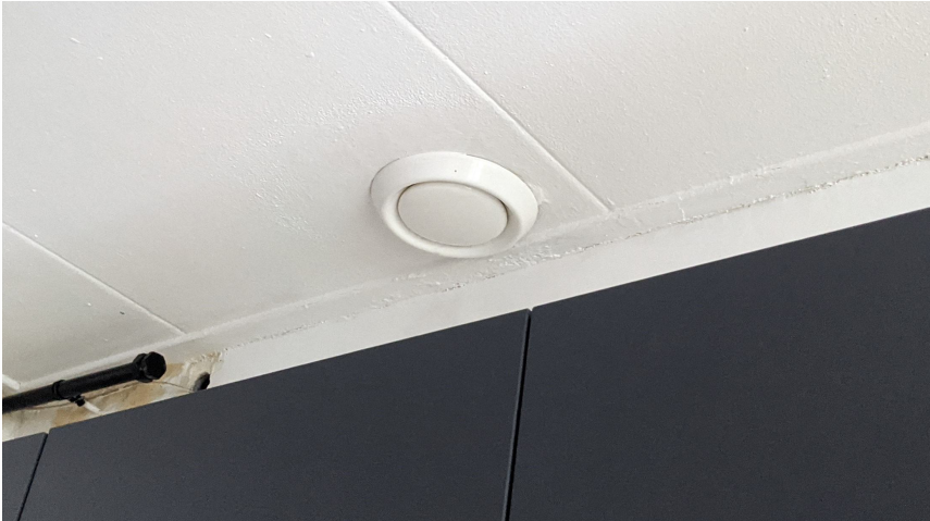
Fig. 30: Exhaust vent above kitchen cabinet
