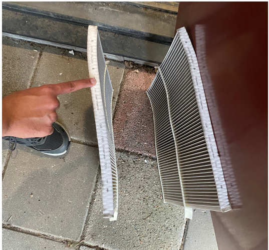
Fig. 119: Both filters are coarse and inserted in the incorrect orientation according to the indicators
