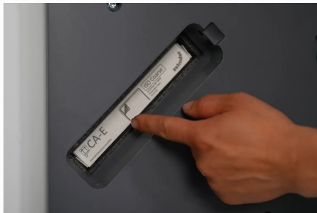
Fig 71: Filter inserted in Zehnder Unit
