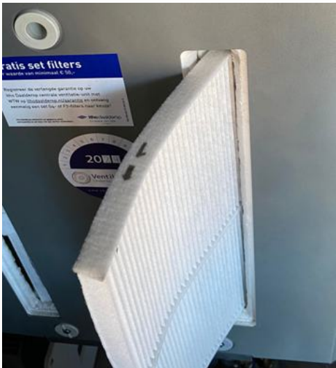
Fig. 118: Filter inserted in the wrong direction
