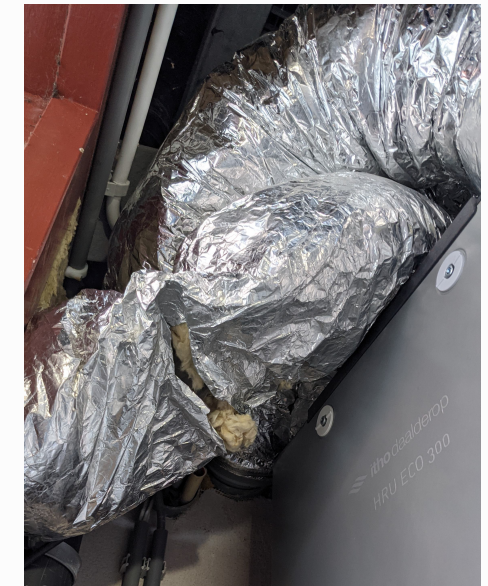
Fig 44: Damaged ventilation unit
