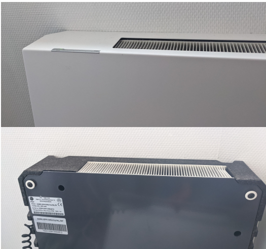
Fig. 27: MV unit with outer cover removed
