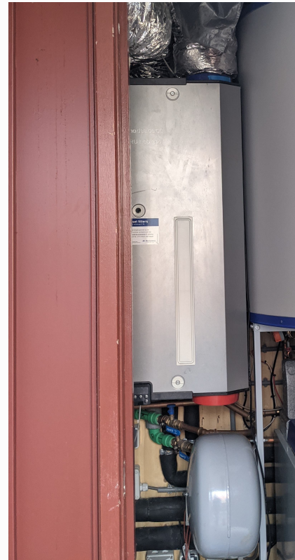
Fig. 34: MVHR Unit placement in skid
