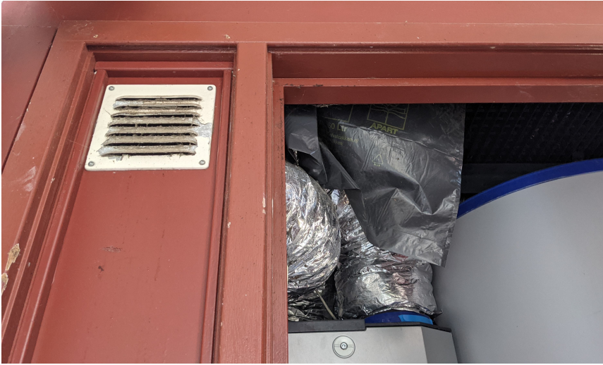
Fig. 31: Inlet vent to skid very dusty
