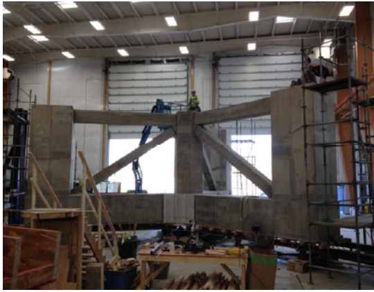
(a) During construction
