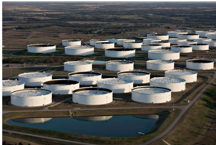
Figure 35: Liquid bulk tanks with external floating roofs. Source: Google
