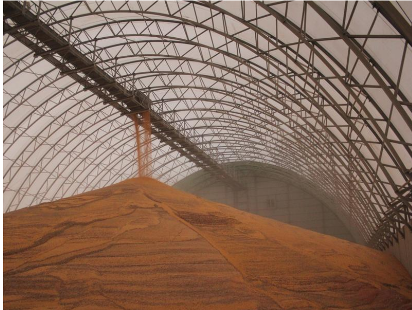
Figure 25: Covered storage with a belt conveyor for stacking. Source: Google
