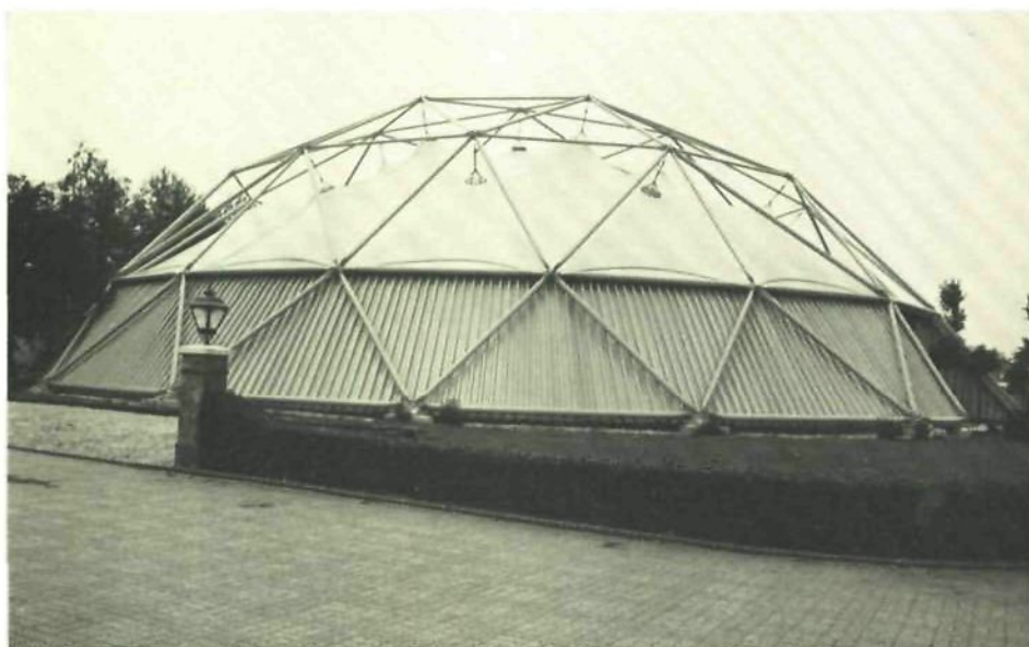
157, 158 The 40 m diameter exhibition dome of the Autotron Car Museum, first built in Drunen (NL) and after 2 years moved to Rosmalen. If required the second membrane can be built on top of the existing one to get a better building physical behaviour.
