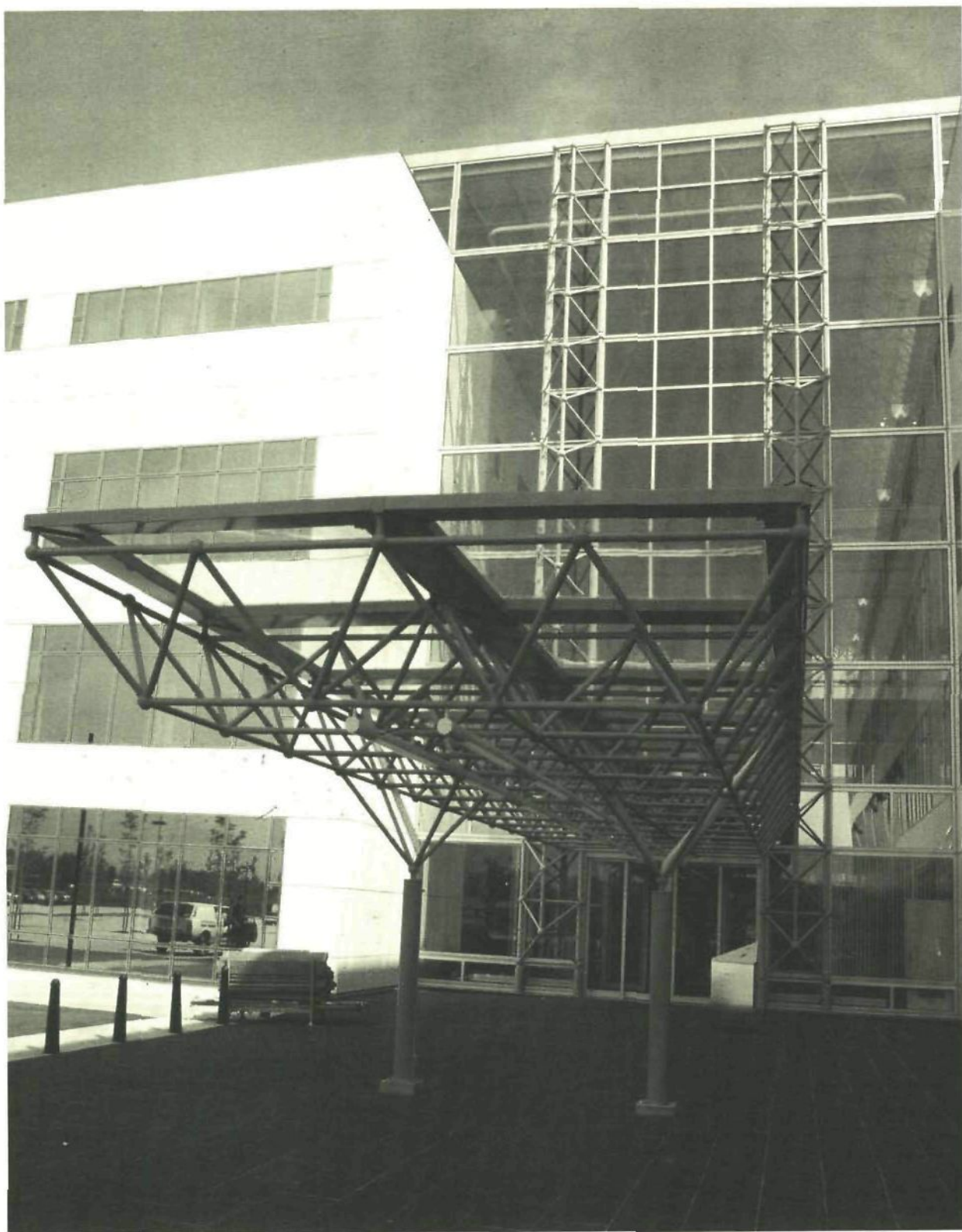
70 Entrance Canopy, Fascia trusses and atrium space frame for the Esso head office Benelux in Breda NL, designed by arch Kraaijvanger. Tuball space frames with welded fascia trusses for torsional rigidity and straightness.
