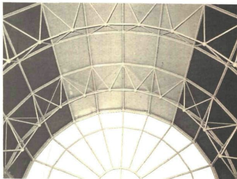
112 Interior views of one of the MRT entrance canopies in Singapore.
