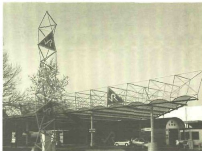
99 Petrol station in Schiedam with suspended translucent covering. (fig 76) Module 3 x 3 m, total size 21 x 45 m, on 5 columns in irregular places of upper and lower chord nodes. Architect John Grootveld.
