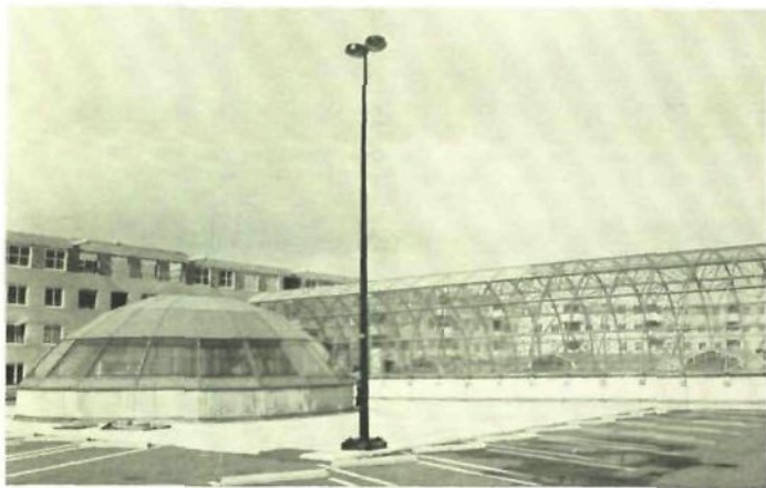
113 Overall view of a shallow 12 m dome partly clad with panels, partly with insulated glass, and the main arcade on the Amsterdam Zuid-Oost shopping centre seen from the first parking floor above the shopping centre. Architect Ben Loerakker.
