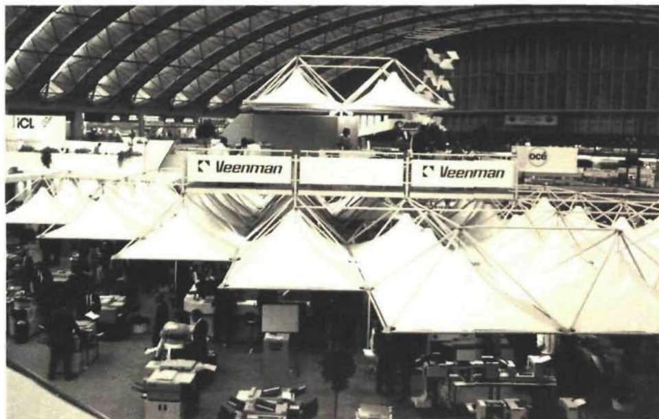
154 Veenman exhibition stand on Efficiency 86 in Amsterdam, consisting of a regular space frame and membrane elements. (fig 81) Architect Frank Pluym.
