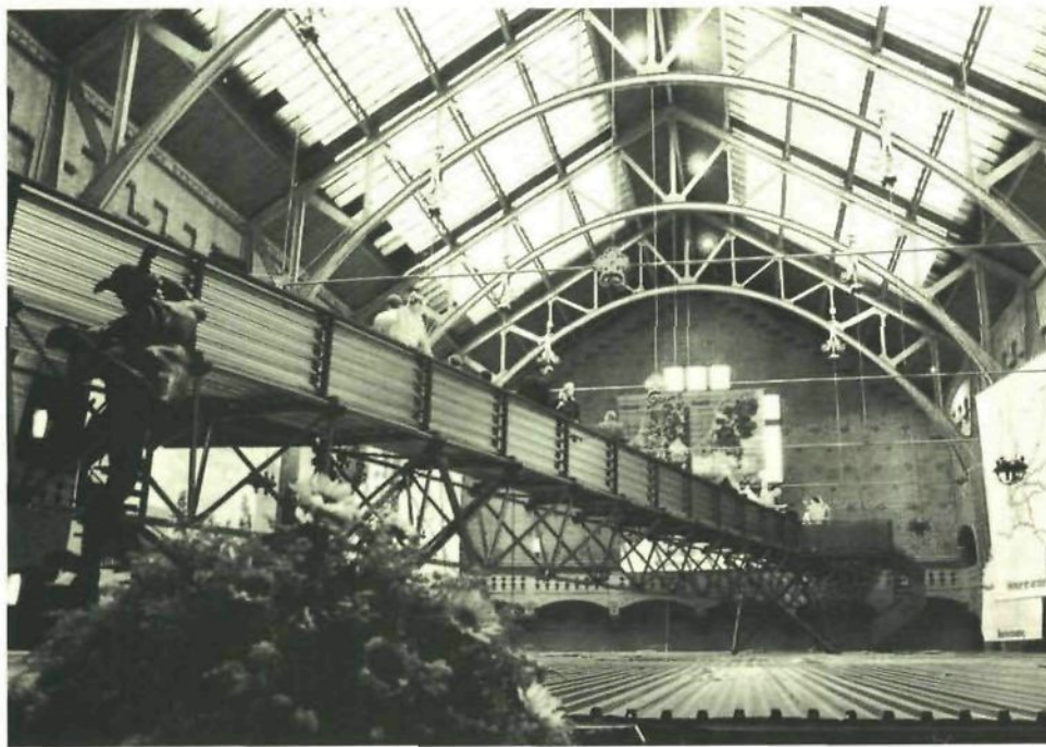
60 The large hall in the famous Exchange of Berlage in Amsterdam during the exposition 'Nederland 2050'. A mezzanine space frame covered with black coated steel panels to accommodate the visual shows on the ground level, with a diagonally crossing space truss bridge at 10 m plus, supported by two tensegrity towers.
