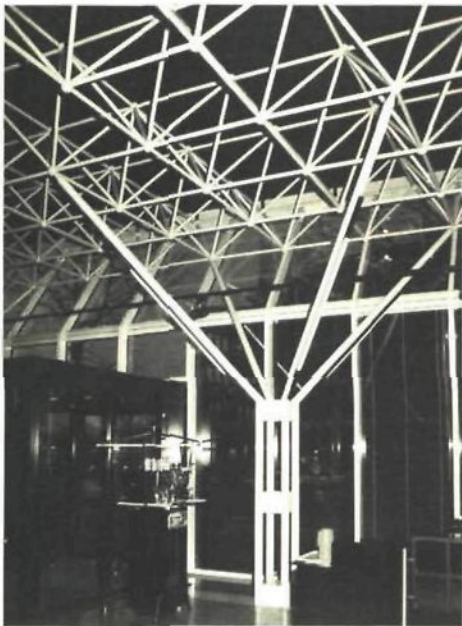
96 Entrance hall for Cap Gemini office, Utrecht supported by 6 tree-like supports. Architect Overhagen.
