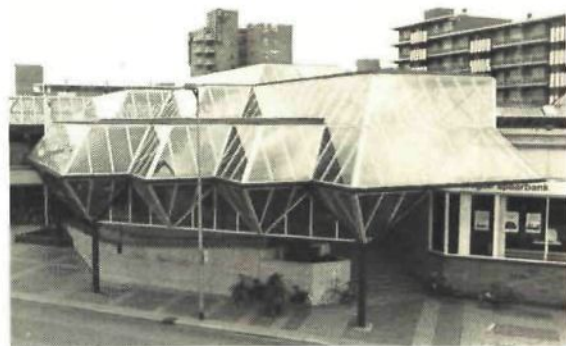
57, 58 The Schollevaar shopping mall with entrance canopies now open to all sides. The glass covering is tightly tailored around the space frame to produce a crystallised form of the multilevel space frame inside. Module of entrance canopies 2,700 m and 1,350 m in the arcades.
