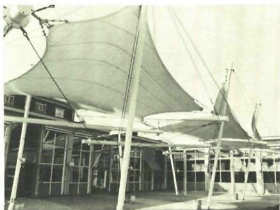
64 The Hemweg Tensegrity Structure. (model in fig 23) Tubular elements not directly connected, only indirectly by cables. Masts dia 160 mm, cables dia 10 to 16 mm galvanised steel. During the winter 3 membranes are stored to remain only a graphical play of white tubes suspended or 'floating' in the air. When during springtime the membranes are installed again an extra outdoor area for the adjacent canteen is available.
