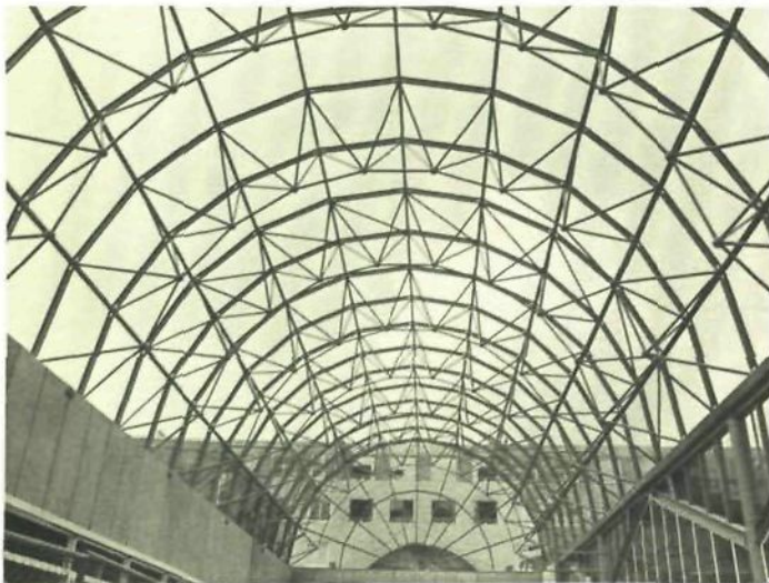
113 Overall view of a shallow 12 m dome partly clad with panels, partly with insulated glass, and the main arcade on the Amsterdam Zuid-Oost shopping centre seen from the first parking floor above the shopping centre. Architect Ben Loerakker.
