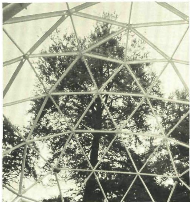
41 Initial design model made by Wiek Röling, consisting of hexagonal and pentagonal faces as a good starting point for further development of the preliminary design.
