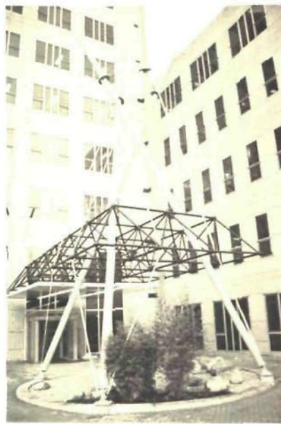
131 Overall picture of the tensegrity canopy for the 'Nederlanden van 1870' office in Diemen (fig 134).
