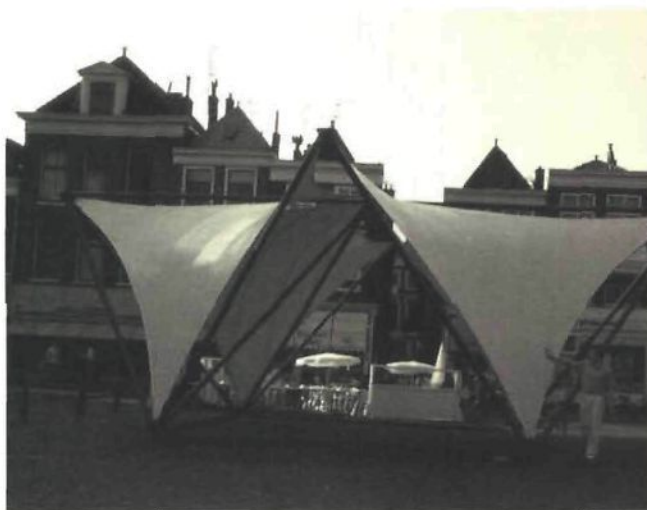
163 Macro space frame in standard 6 m Octatube with 4 separate prestressed membranes for an exhibition stand for Modulex, Hoofddorp (NL), designed and realised 1986 by industrial designer Rogier de la Rive Box and the author.
