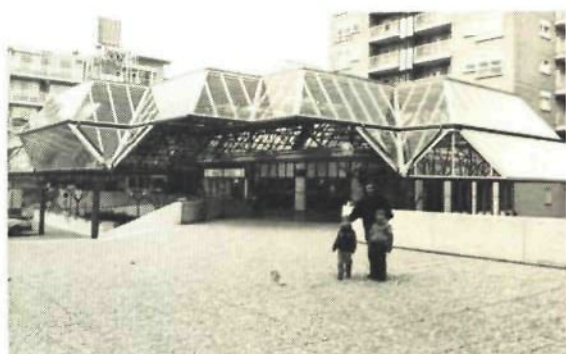
56 Bird's eye view of the original space frame covering for the Schollevaar shopping mall in Capelle a/d IJssel showing the sculptural open space frame elements. In a second design and building phase, started after inauguration of the shopping centre, a complete covering was realised. See fig 103 after realisation.
