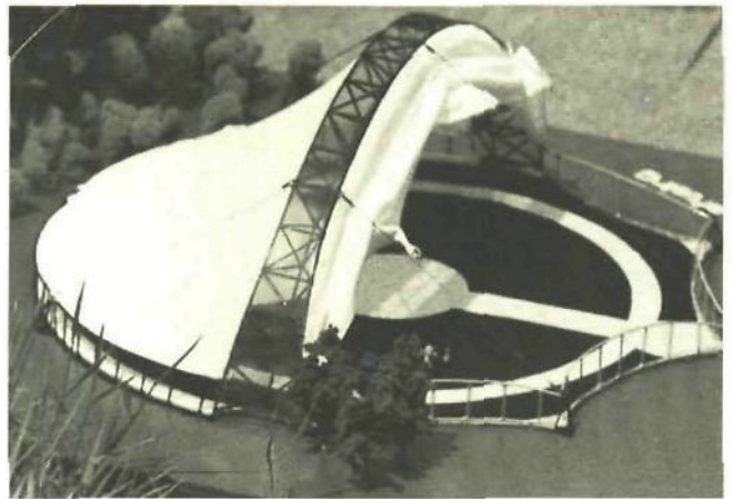
141 Model of movable tent roof for leisure park 'De Efteling' in Kaatsheuvel NL. Height arch. 25 m., span 60 m. ground plan E 60 m. diameter (not realised)
