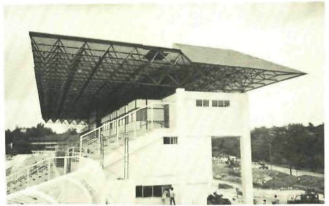
68 Picture of the first Octatube space frame as a grandstand covering, cantilevering 18 m, on a total length of 70 m, over a stadium in Kuala Lumpur. Engineering was done in Delft, manufacturing and installation done locally by Octatube Malaysia, 1988.
