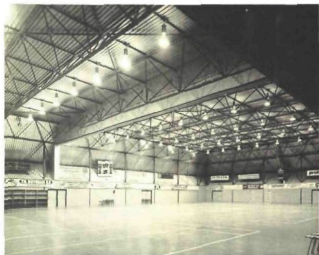
107 Interior of the Quintus sporting hall in Kwintshuyl NL, showing independent space trusses with separate wind bracing in the upper chord plane. The light armatures are chosen in a non-directional way, in order not to conflict with the squareness of the space frame modules. Architect author, 1978.
