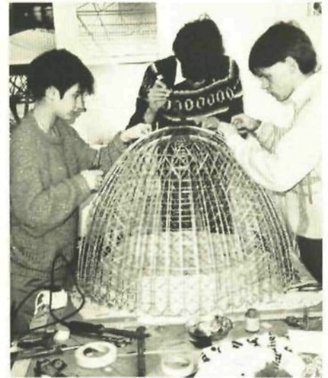
125 Soldering of the model took about four weeks with three to four designers (1987). Computer drafting of the presentation drawings two days and one engineer.
