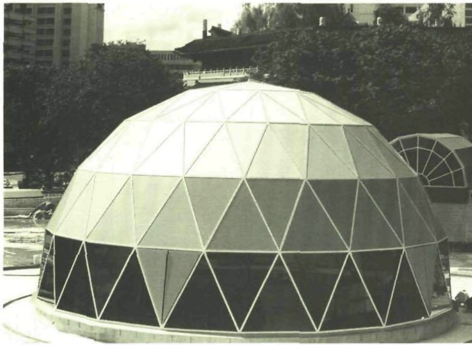
118, 119, 120 Overall view, interior and details of the main dome dia 15.5 m over the Orchard Boulevard MRT station in Singapore, clad with aluminium sandwich panels/insulated glass panels. The five lower panels are 4 double smoke exhausts hinged on both sides and one service door, hinged on the upper side. All elements have been detailed with an internally surrounding welded steel gutter with details; working like a car door type 'hatch back'.
