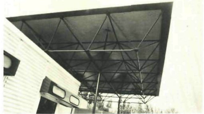
153 Space frame and stretched membrane on top for an entrance canopy of a storage building in Oegstgeest. Architect Jan Brouwer 1983
