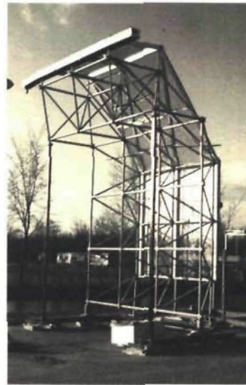
26 Performance tests by TNO Delft for static and dynamic over- and underpressure combined with water spray tests for watertightness of a skylight system for the Raffles City Complex skylights in Singapore 1984.
