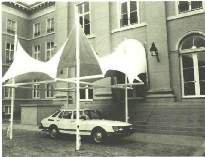
142 Temporarily entrance canopy for the palace of Her Majesty the Queen of the Netherlands in The Hague. This structure is only installed for reception of official guests.
