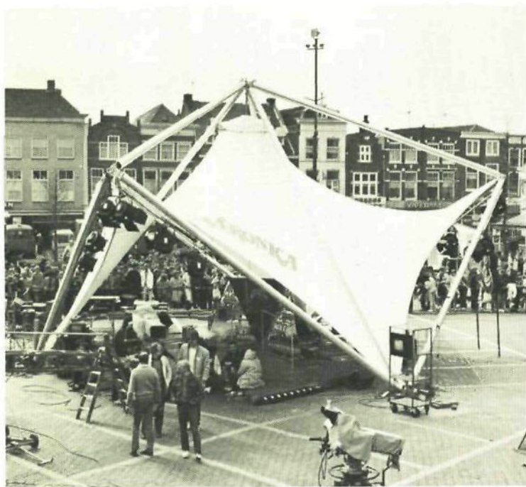
63 The Veronica Music Tent, in use every two weeks during the season at changing locations since 1982. Composed of a macro space frame in galvanised tubes dia 160 mm with lengths of 9 to 11 m, with a suspended prestressed membrane, calculated to resist windforces up to Beaufort scale 10.
