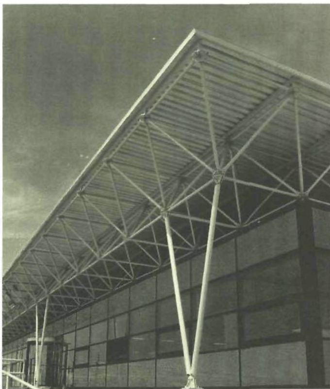
93 Customs office building in Hazeldonk (NL-B) in Octatube with a single aluminium roof decking on top, and insulated roof panels suspended to form a free office space. Total plan size 17 x 68 m, module 1.8 m, depth 1.2 m. Geometry delta trusses with a double fascia delta truss. Architects Benthem and Crouwel.
