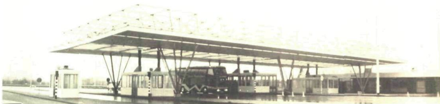
35, 36 Customs border station in Nieuweschen, designed by architects Benthem and Crouwel. Erection over an existing and still functioning expressway took place during the night, after assembly on an adjacent parking ground, transport in two parts on a 64-wheeled trailer and hoisted by mobile cranes. Size 24 x 51 m, module 3 x 3 m, depth 2.1 m.
