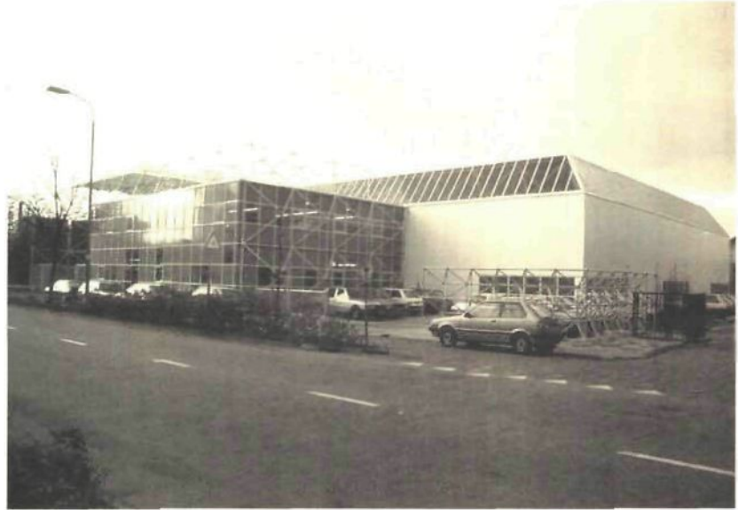
97 Tuball space frames around the main Octatube office in Delft. Size 12 x 30 m in plan. The frame carries the roof level of the first floor plus the sun shading tent structure on top. Architect author. (1985)
