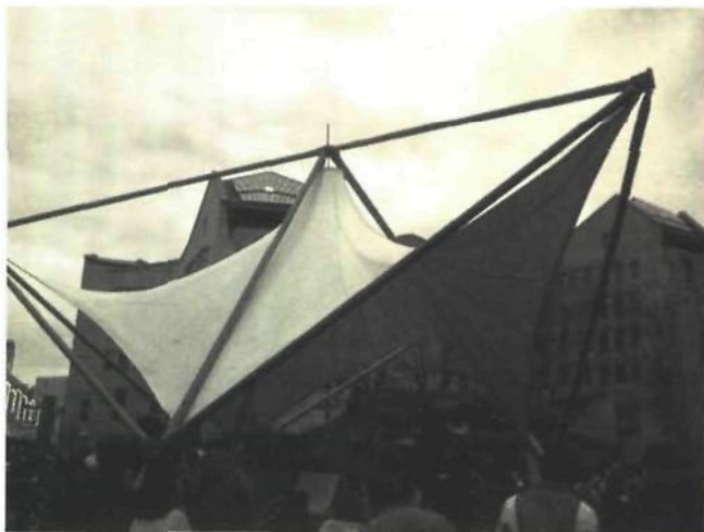
162 Standard 6 m module aluminium macro-space frame with internally prestressed membrane, complete with a triangular space frame stage platform with plywood boarding, for the shopping centre Amsterdam Zuid-Oost, (1987). Design author.
