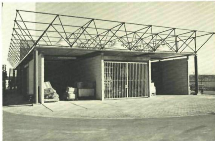
156 First large scale application of a regular Octatube space frame 21 x 42 m realised in 1988 for Beyersdorf in Almere (NL). Architect Op ten Noord/ Blijdensteyn.
