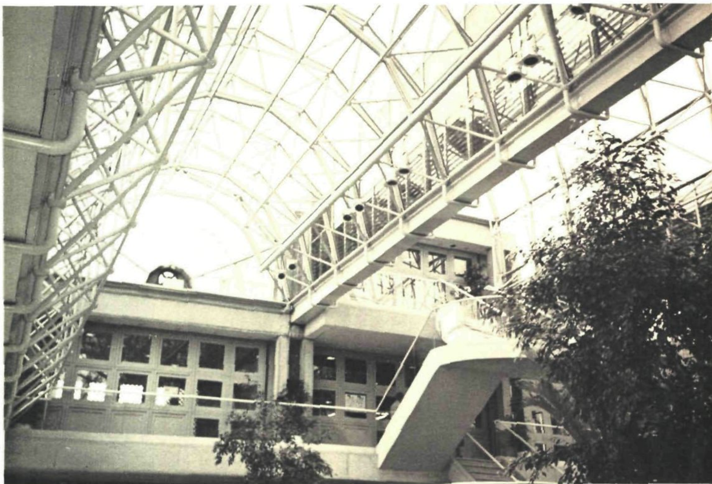
49 Interior picture of the Serangoon Atrium.
