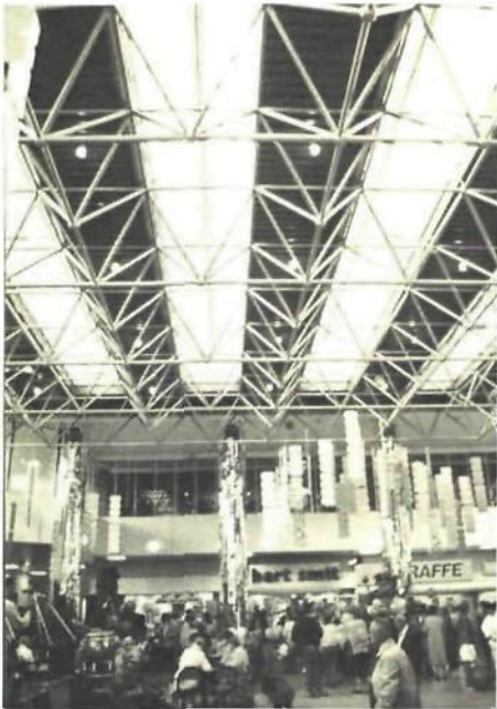
95 Tuball space frames for shopping centre De Klanderij in Enschede (NL) in metallic grey. Architect Spruyt, De Jong, Heringa.
