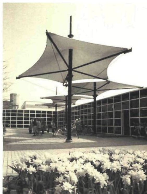
67 Final realisation of 4 lily-like tent elements, consisting of poles dia 300 mm (7 m high), bracings dia 100 mm and tensile bars dia 10 mm, as a result of the respective material efficiency in bending, compression and tension.
