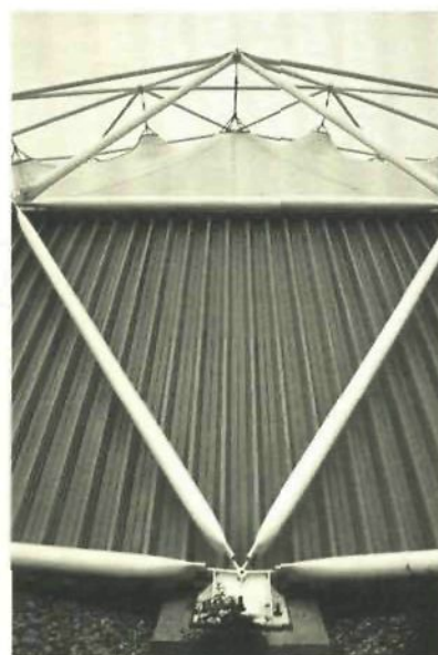
157, 158 The 40 m diameter exhibition dome of the Autotron Car Museum, first built in Drunen (NL) and after 2 years moved to Rosmalen. If required the second membrane can be built on top of the existing one to get a better building physical behaviour.
