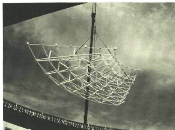
59 Erection of a space frame in the plan form of a quarter circle for the town hall of Huizen (NL) in 1985. Only during hoisting this structure was really a 'Space Structure' in all meanings of the word.
