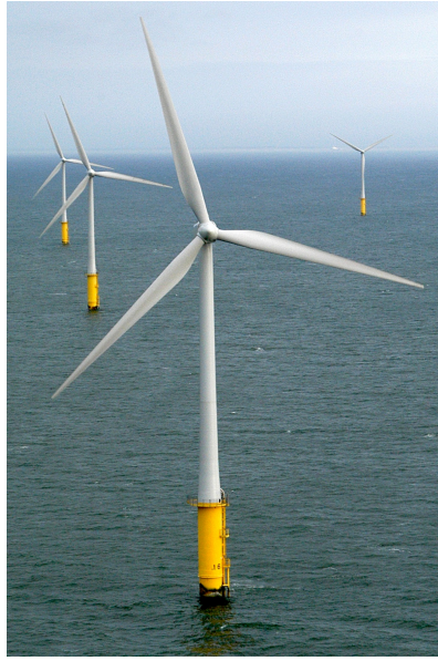
(a) Vestas V80-2.0MW wind turbine at North Hoyle (UK) wind farm (Vestas Wind Systems A/S, n.d.).
