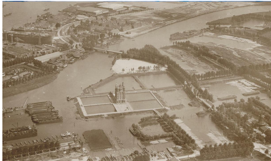
Aerial photograph of Watertorenterrein (RegionaalArchiefDordrecht, 1920).
