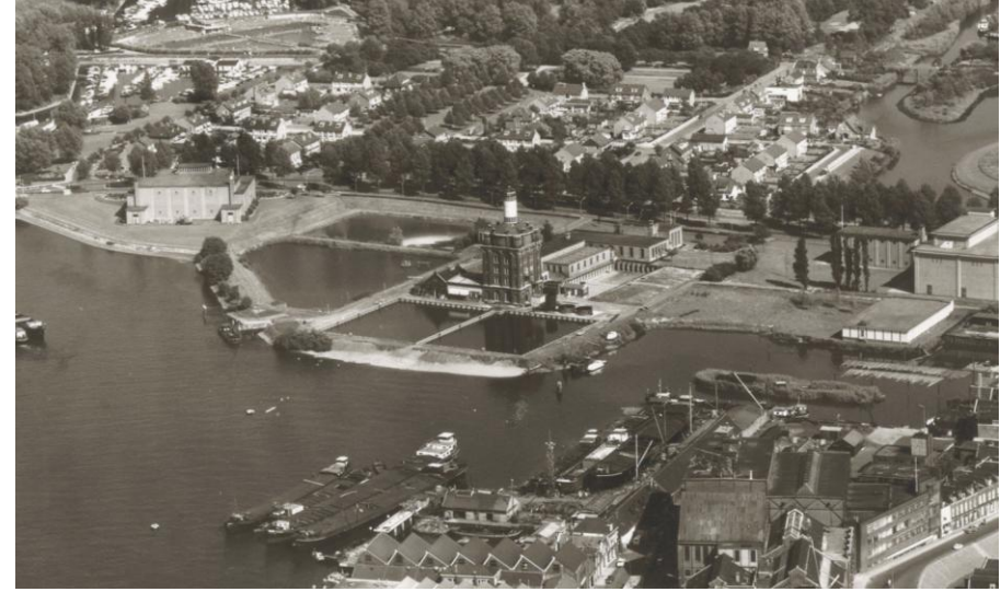
Aerial photograph of Watertorenterrein (RegionaalArchiefDordrecht, 1964).
