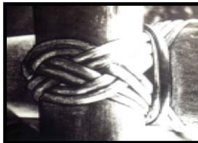
Joint with rattan lashing (Dunkelberg 1985)
