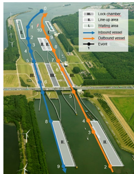
Figure 1 The Volkerak lock complex with highlighted infrastructural elements that are critical for modelling the vessel behaviour (logistics) during lock passages. Critical elements and events are numbered (image by F.P. Bakker & M. van Koningsveld, is licenced under CC BY-SA 4.0, the background image was retrieved from https://beeldbank.rws.nl , Rijkswaterstaat).
