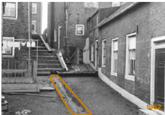
figure 17: Water drainage on the streetsurface, already implemented in the so called 'stoepen' in Sliedrecht (left). (Left: Historische Vereniging Sliedrecht, 1962. Edited by my own. Right: Pötz & STOWA, 2014)
