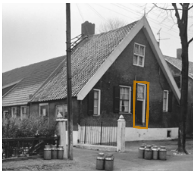
figure 14: Barn in Alblasterdam with a higher flooddoor (VVV Alblasterwaard, n.d. Edited by my own)
