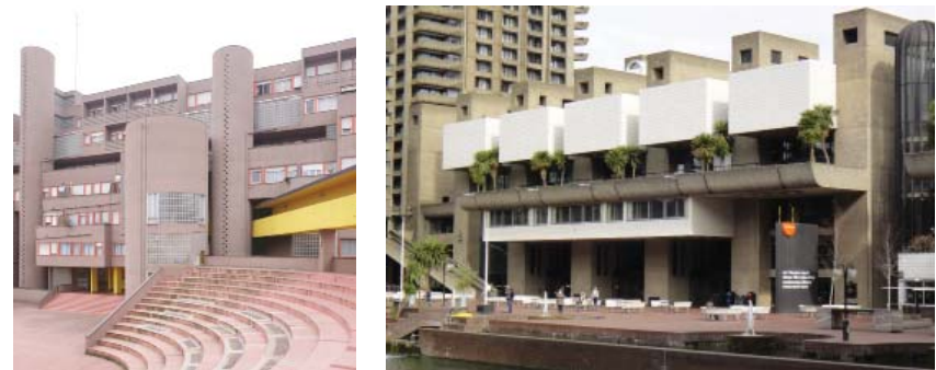
Left: The bright yellow indicates the circulation areas (Gallaratese, Milan) Right: The white tiled elements indicate the public function of the building (Barbican, London)
