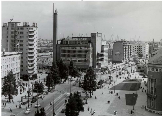
1950 - depart partly destroyed building bijenkorf for Beurs
