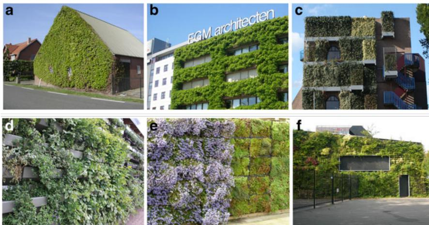
**Figure 5.8:** Vertical greening systems: Direct greening system (a), indirect greening system (b), indirect greening system combined with planter boxes (c), LWS based on planter boxes (d), LWS based on foam substrate (e), LWS based on felt layers (f) (Perini et al., 2013)
