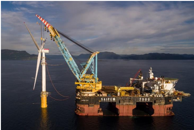
Figure 13 Saipem 7000 twin-lift fully assembled wind turbine installation (Saipem, n.d.)
