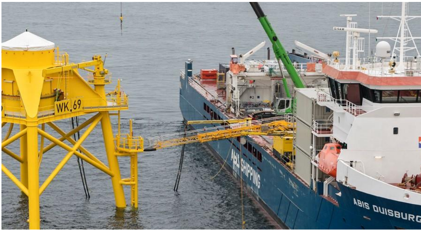
Figure 37 Gangway to access wind turbine (SMST, n.d.)
