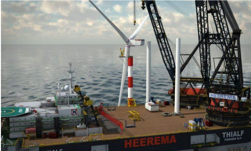
Figure 16 Heerema Thialf wind turbine installation method using dummy tower (Tacx, 2019)
