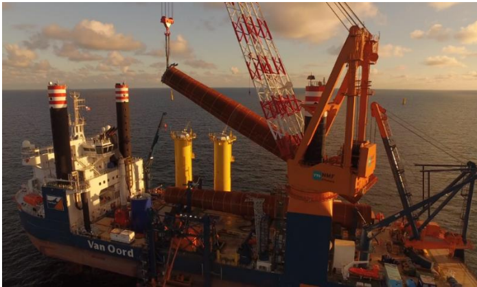
Figure 26 Monopile upending by Van Oord Aeolus Jack-up vessel (Van Oord, 2016)
