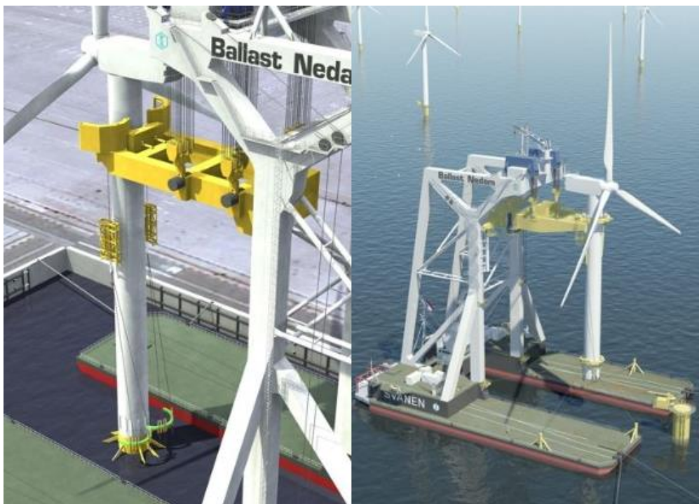
Figure 15 Svanen with special adapter to install wind turbines (Wermeskerken, 2013, slide 11)
