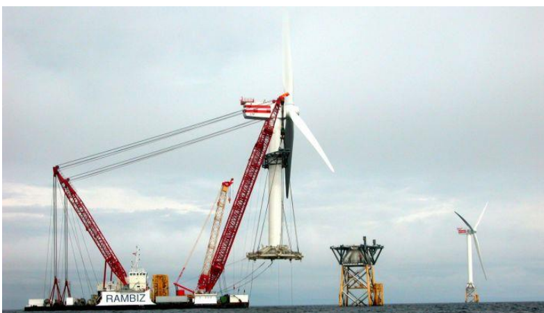
Figure 12 Rambiz floating crane installing wind turbine (Huisman, n.d.b)
