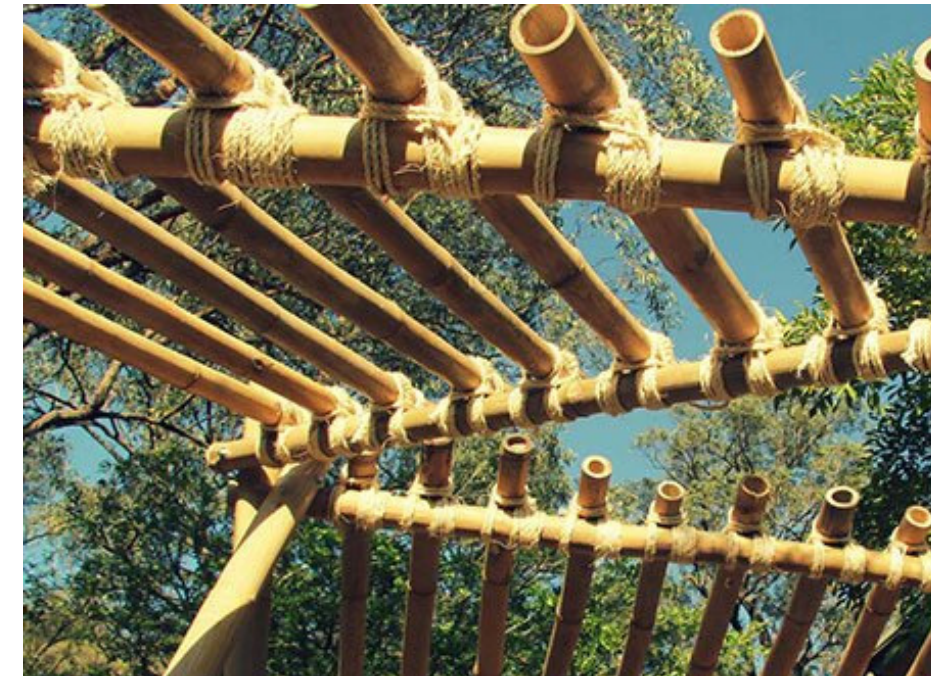
figure 61: bamboo joining technique: Lashing 103
