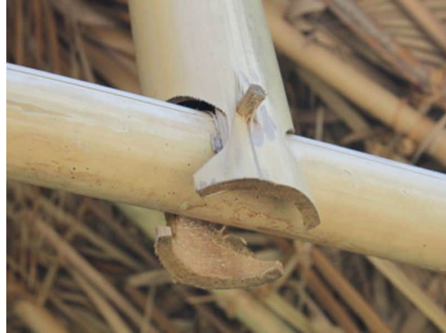
figure 60: bamboo joining technique: Mortise and tenon 104
