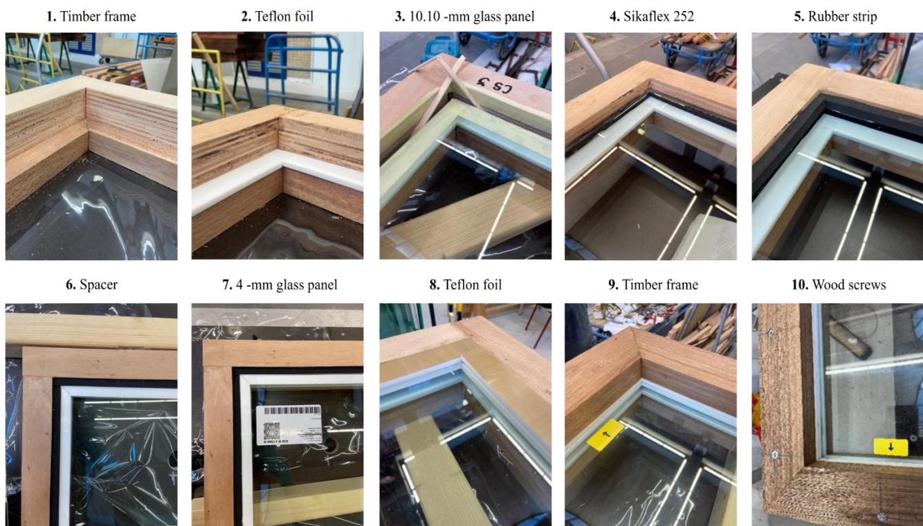
**Figure 2.** Overview of the structural glass window construction.
