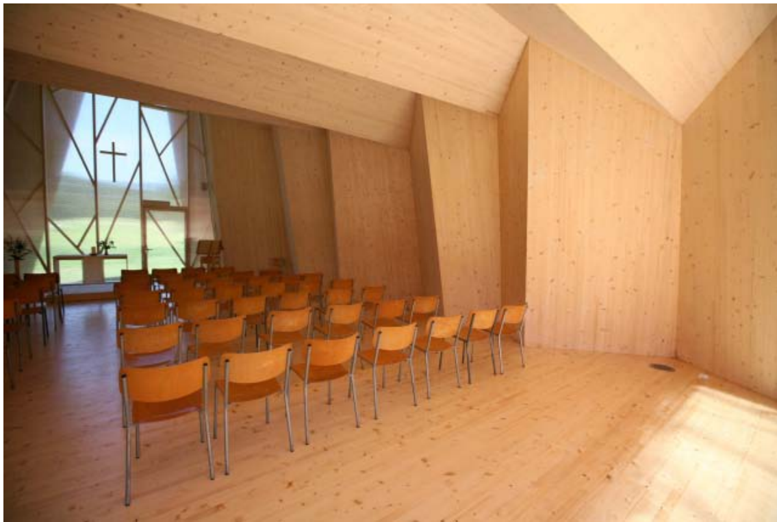
Fig. 4: Origami structure in CLT as temporary chapel in St. Loup, Switzerland
