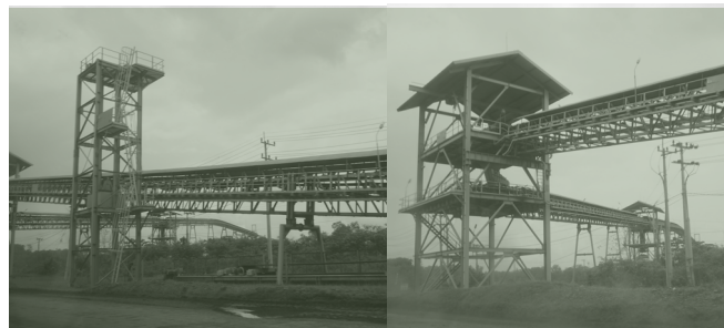
Transport tower & Conveyor system
