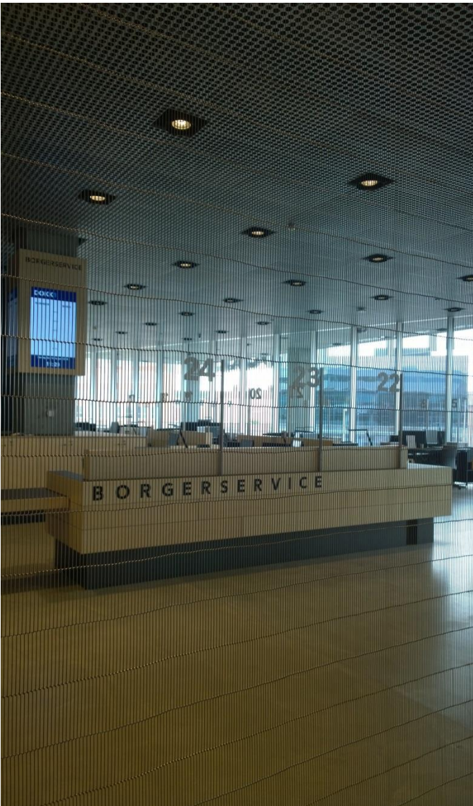
Fig. 8: Separation with steel wired 'curtain' (own photo)
