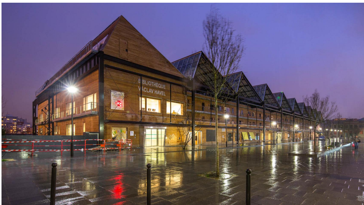
Fig. 2: La Halle Pajol; old structure welcomes new wooden building
