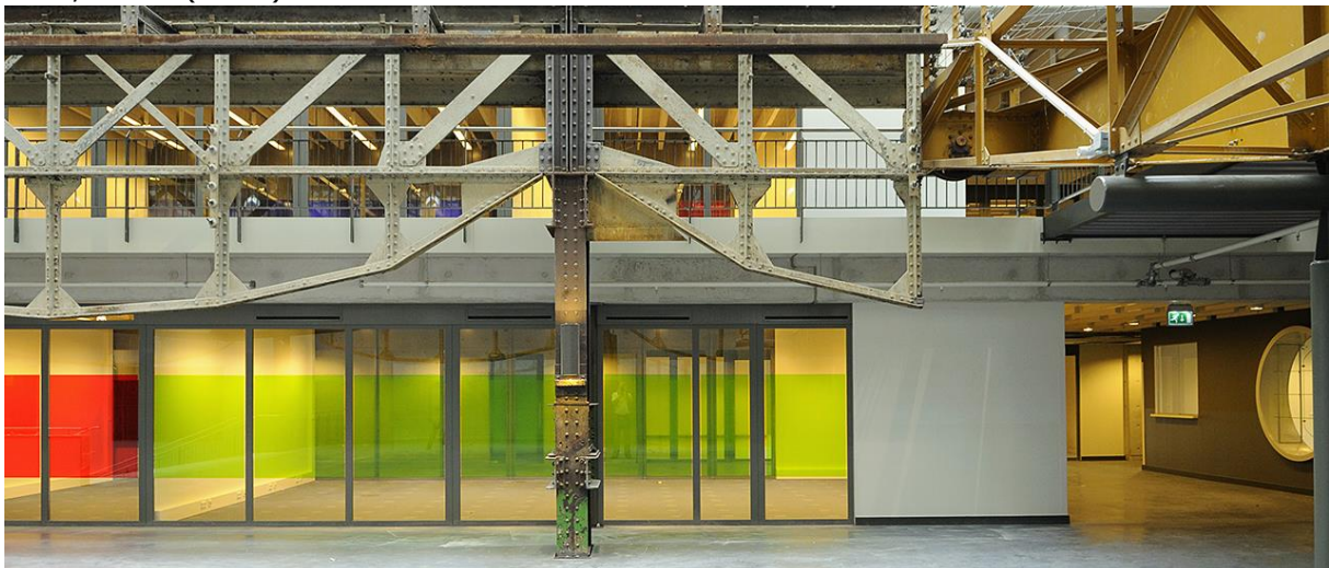
Fig. 12: construction of old hall and new building parts
