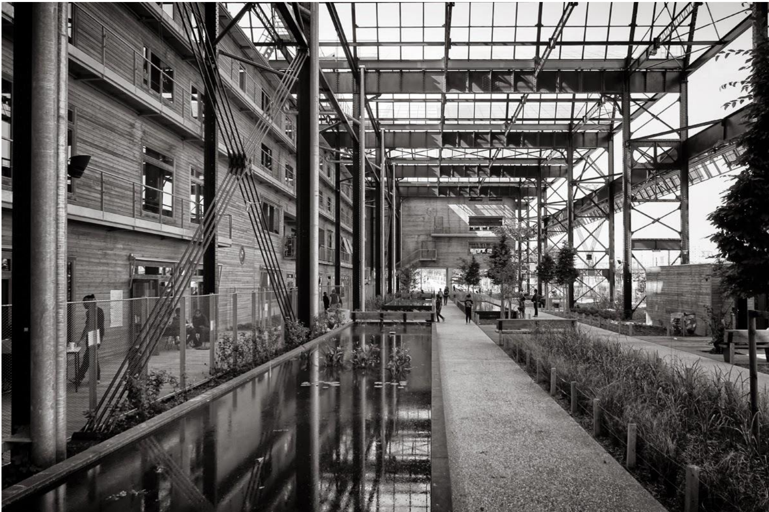
Fig. 3: La Halle Pajol; covered public garden as interior space. Refurbished and cleaned up steel structure creates new atmosphere.
