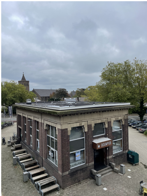
(a) Top view photo 1 of Bouwpub
