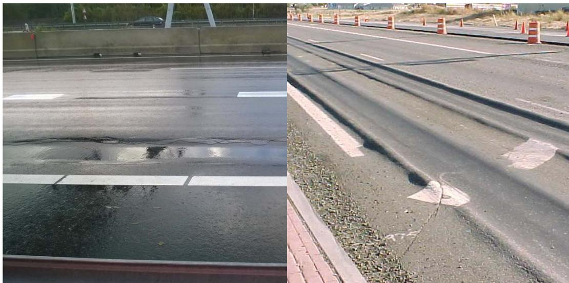
Picture 3.3 Rutting due to weak subgrade (left), and rutting due to weak asphalt layer [10] (right)
