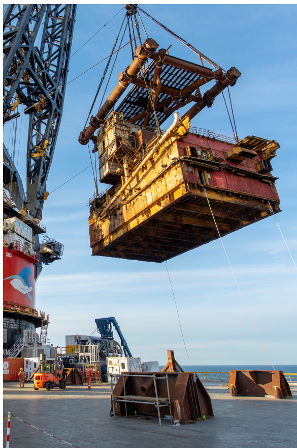
(a) Grillage beams on deck
