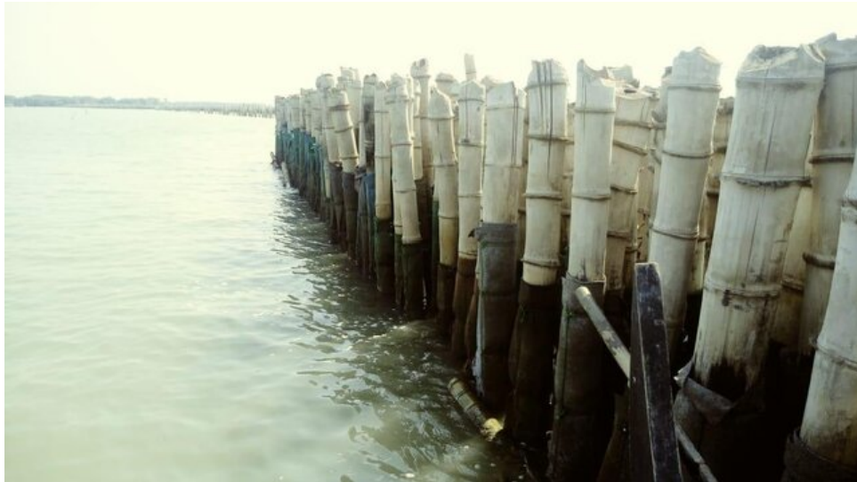
Figure 4.5: An application example of using a bamboo breakwater (Achiari et al., 2020)
