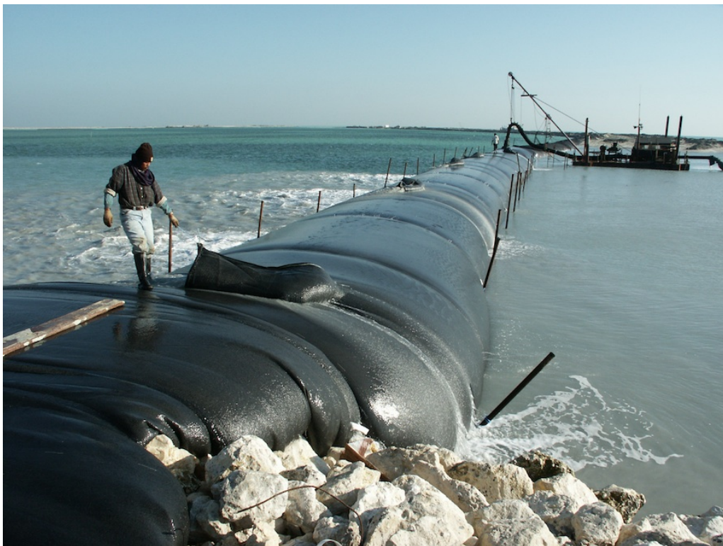
Figure 4.4: An application example of using a geotextile tube breakwater (Ocean Global, 2022)
