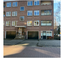
Figure. Parking box entrance disrupting sidewalk
