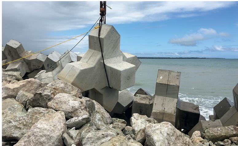
Figure 1.3: Xbloc placement on a breakwater
