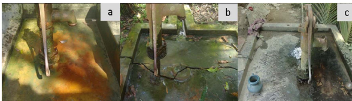
Fig. 5. Typical colors developed on the platforms of the tubewells a) Red; b) non identified (NI); and c) Black. (For interpretation of the references to color in this figure legend, the reader is referred to the web version of this article).
