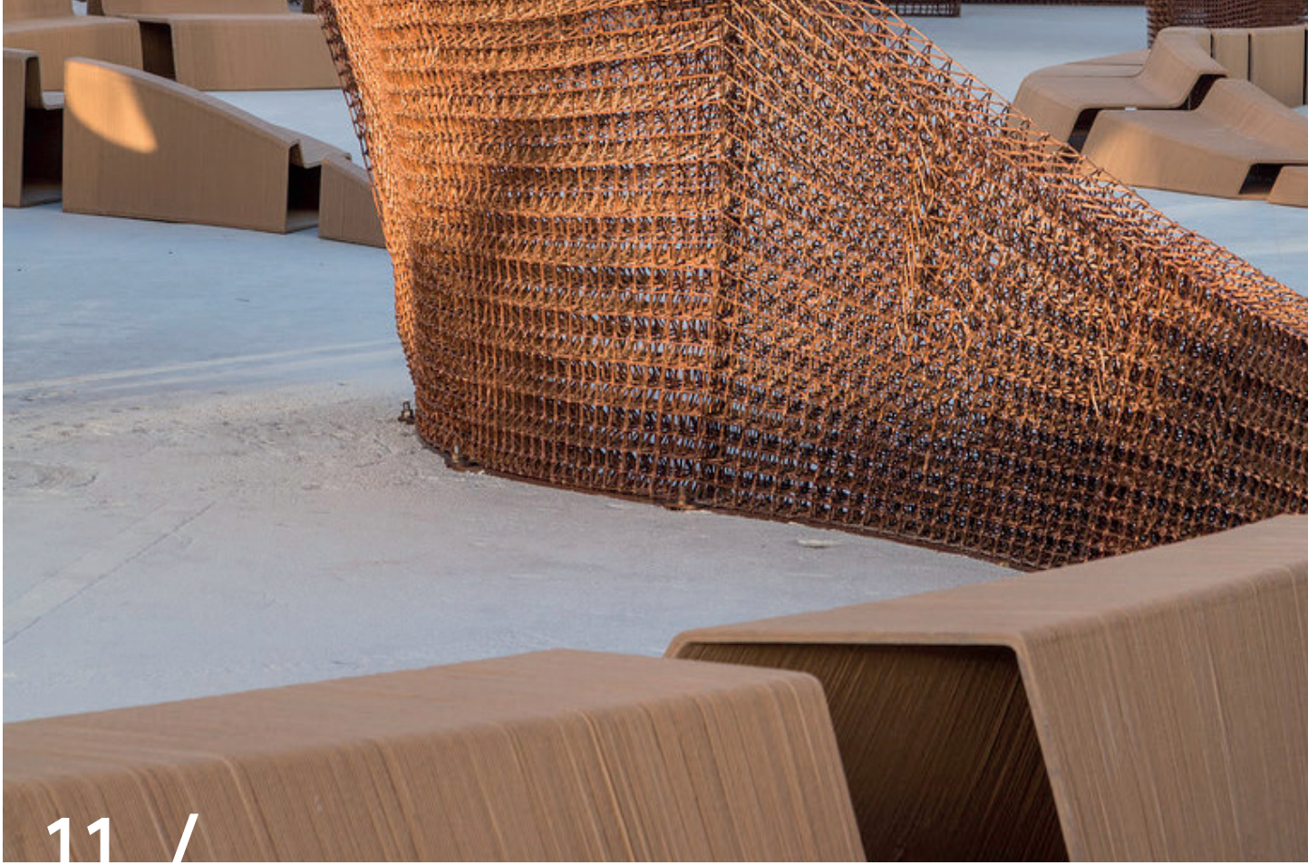
Figure 11: Flotsam & Jetsam/ ▶ 3D printed bar and benches from bamboo reinforced PLA. (Produced by: Oak Ridge National Laboratory)
