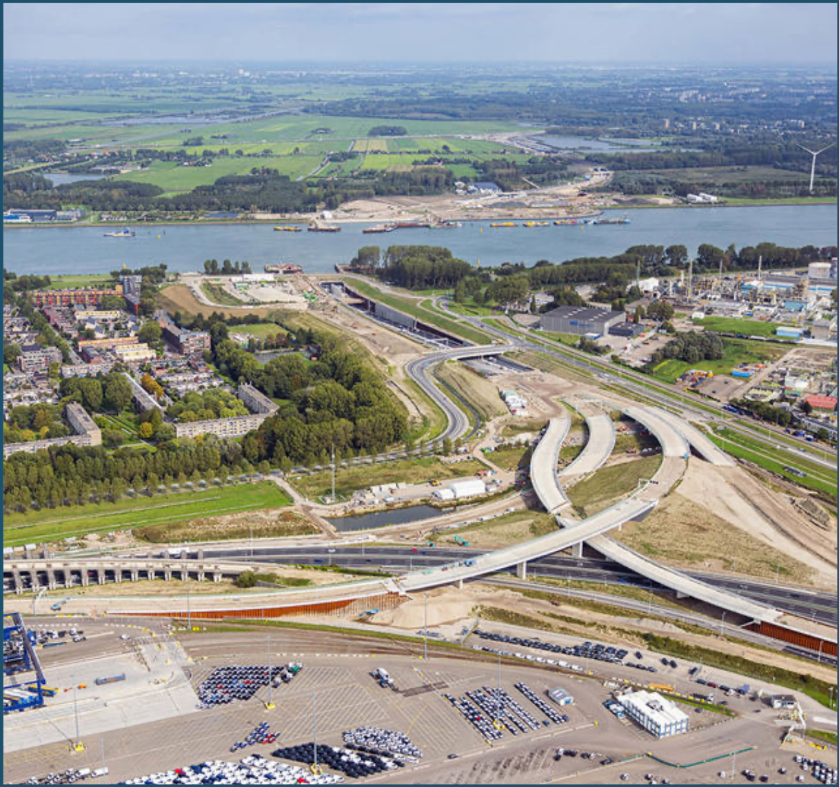
Figure 12 Image Case2. Ballast Nedam (2022).
